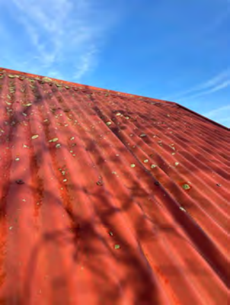
Example of lichen growth on the roof cladding.
