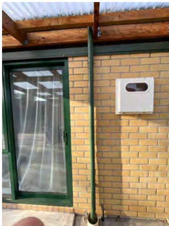
Example of rusting gutters and down pipes needing replaced and or repaired.
