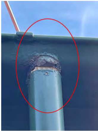
Example of rusting gutters and down pipes needing replaced and or repaired.
