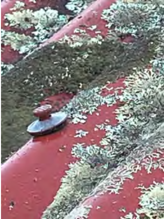
Example of roof fixings that has popped.
