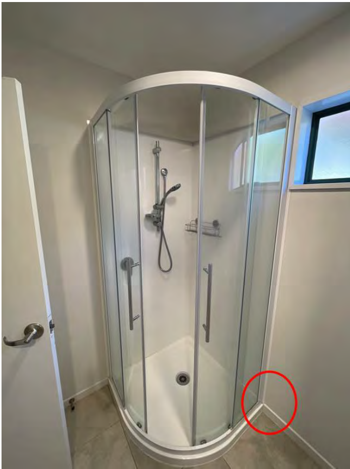
Small leak in this corner and a leaky shower head which may require tightening.
