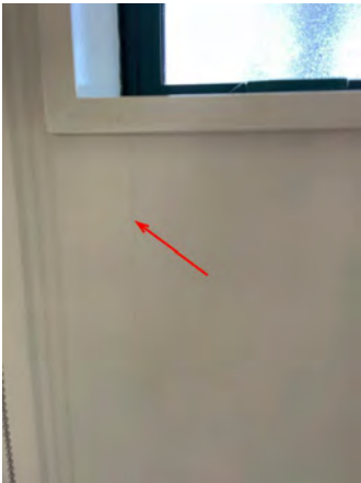
Example of minor crack in the plasterboard. NW bedroom.
