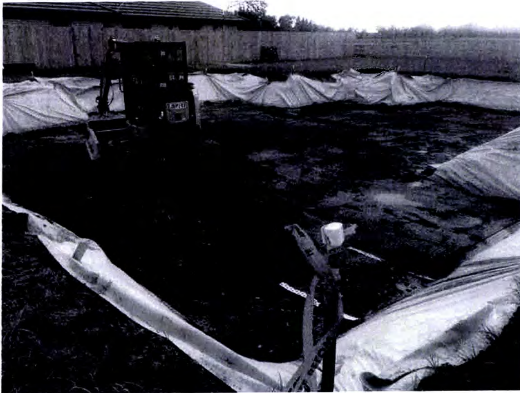
Photograph 1) General view excavation undertaken to date with the first lift of hardfill and the first layer of geogrid placed
