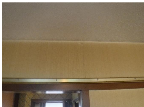
Photo 9. Cracking damage to the internal wall linings (Unit -1).
