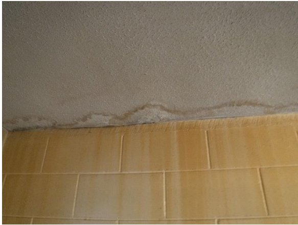
Photo 10. Water ingress identified to the unit 2.
