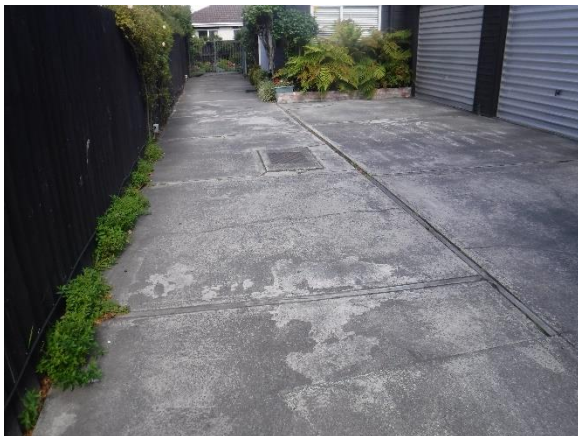
Photo 6. Cracking damage to the concrete driveway.
