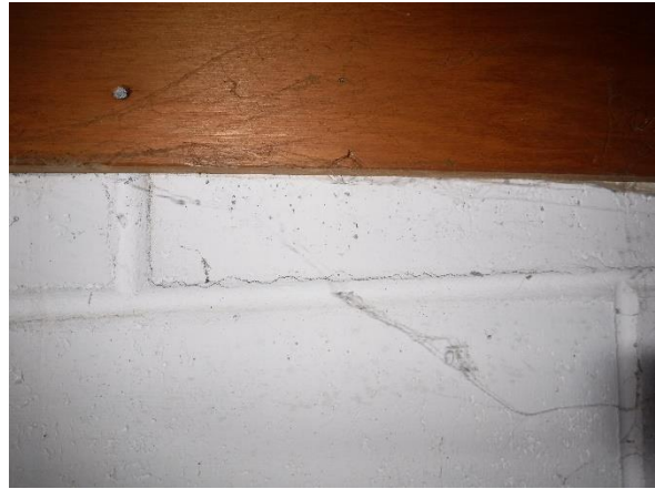
Photo 11. Minor step cracking to the block wall.
