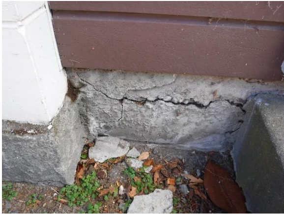
Photo 4. Cracking damage to the concrete perimeter foundation.
