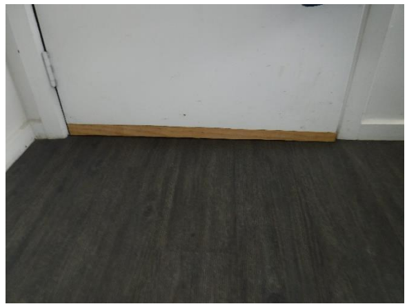
Photo 13. Door misalignment view 2 (Unit -2).
