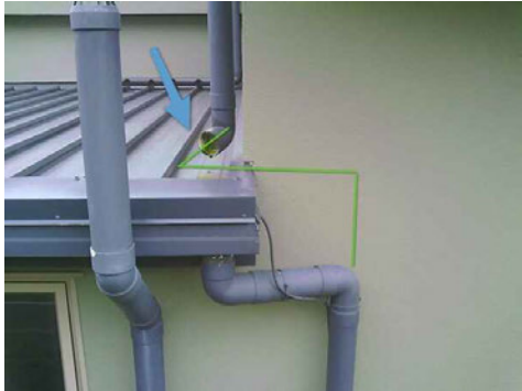
Modification to downpipe has now been made
