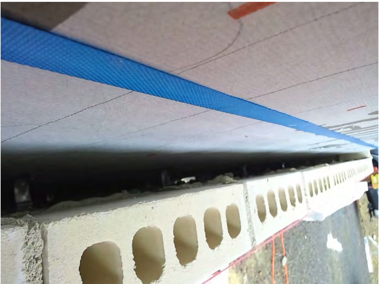
40mm cavity and brick ties
