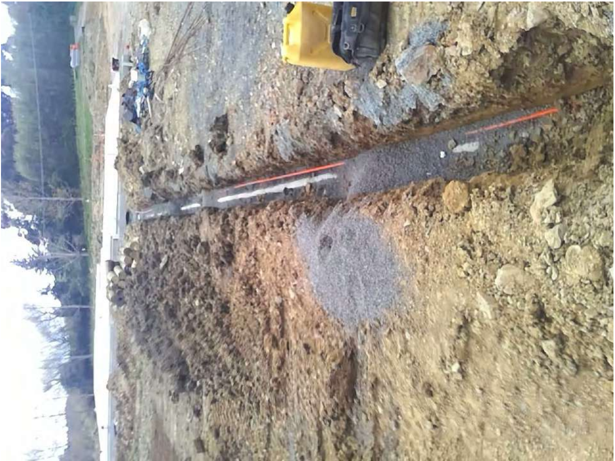
Sewer drain to septic system Taken at 11:35 AM on Thursday 10/10/2019
