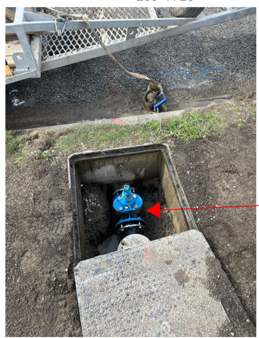
Image 1 - Recently installed Valve and vacuum point
