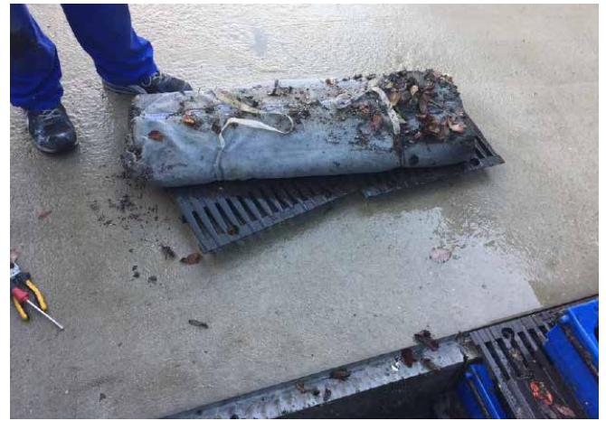
Figure 14. Exchanging the filter bag
