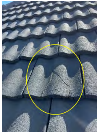
Example of repaired tiles.
