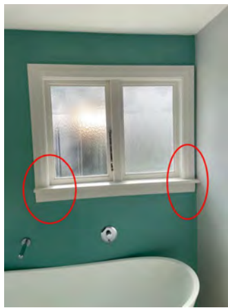
There were two elevated wet moisture readings in the bathroom noted which could be from condensation buildup in the corners of the timber window reveals and sill. This should be further investigated to determine the cause and make good.
