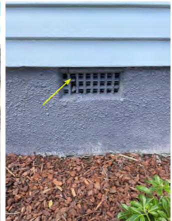
Crack in the foundation vents noted. South face.
