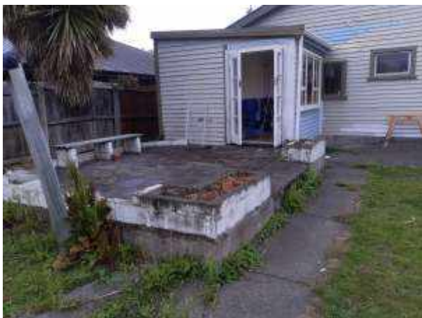
The extension and concrete deck
