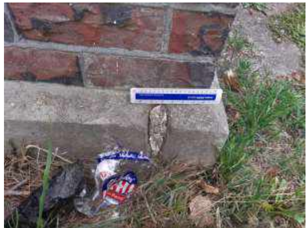
Repaired crack on the porch
