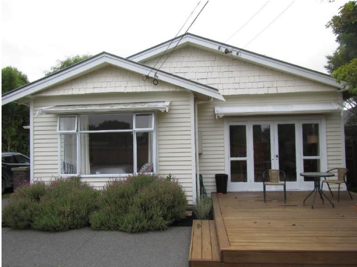
Figure 1: West elevation; deck added and paving constructed since the earthquakes.
