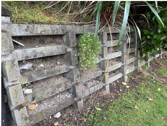
Concrete crib walls are showing no evidence of movement or deterioration
