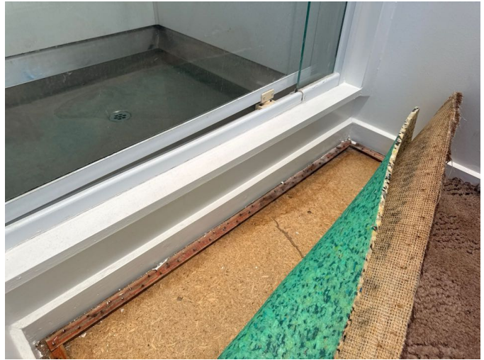
Minor moisture staining at the shower base. The carpet should be replaced with a more durable floor covering.
