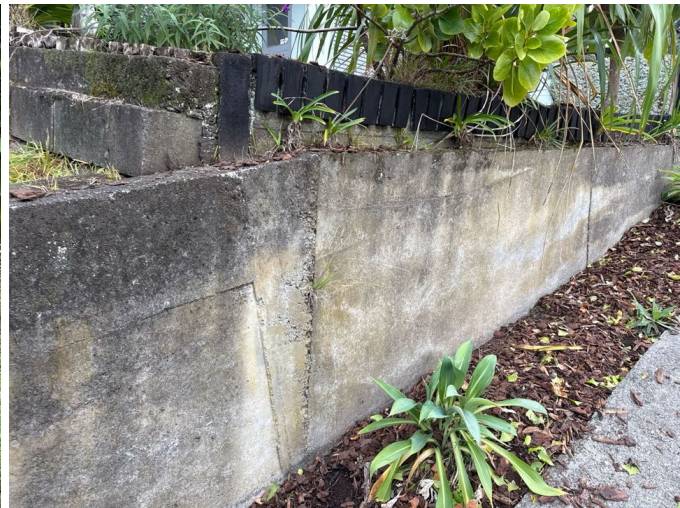
Concrete walls are showing no evidence of movement or deterioration
