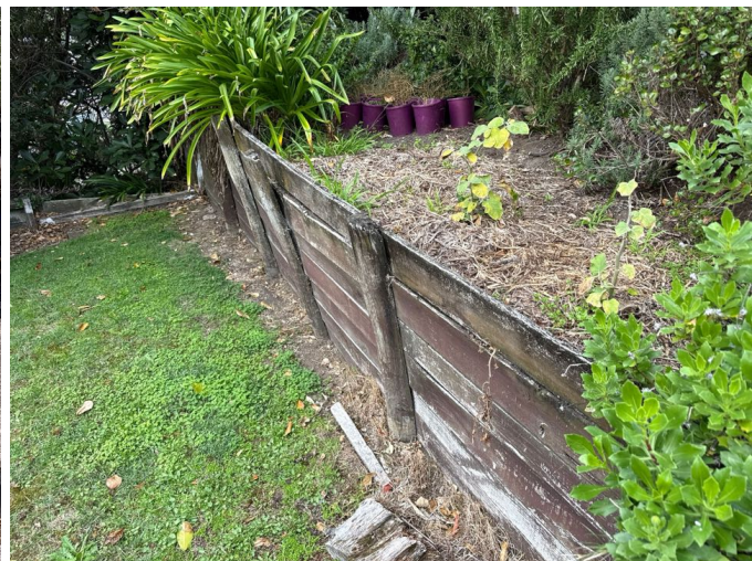
Retaining walls that are leaning significantly at the front should be replaced to prevent the risk of eventual failure.
