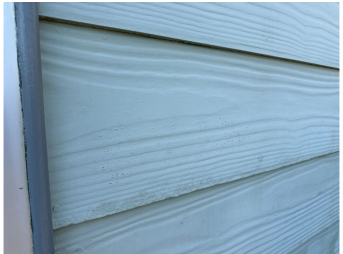
Early stage paint deterioration to the weatherboards
