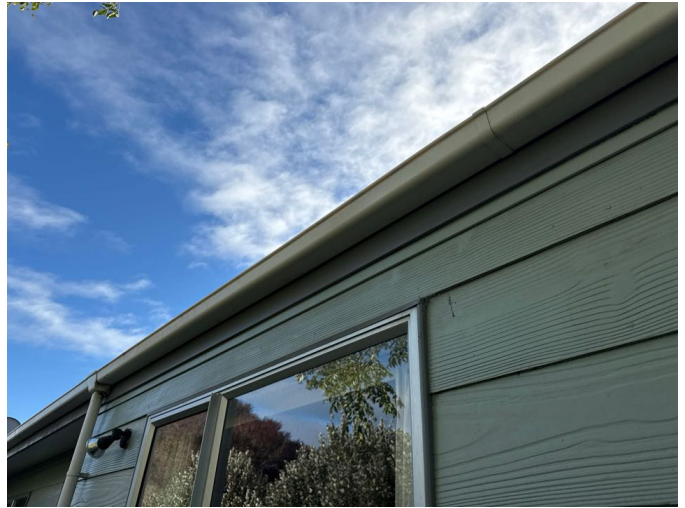
Roof sections where there are no soffits are a higher weather tightness risk. Soffits provide more weather protection to the walls. These areas must be kept in good condition and sealed well to prevent the possibility of moisture ingress. Any failure here has the potential to spill over the top of the wall to the inside of the home. Note there are no current issues here, this is something to watch out for over time.
