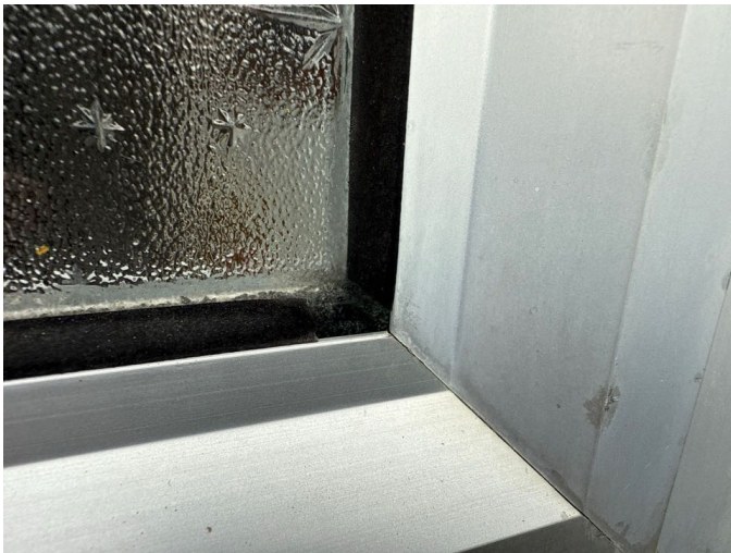
Some of the joinery seals have shrunk which is common for their age. The shrinking seals should not be a water tightness risk as long as the internal seal remains intact and effective. All internal moisture readings taken beneath the windows and doors were within the normal range.
