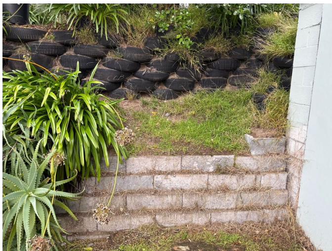
Earth filled concrete block and tyre retaining walls are still effective
