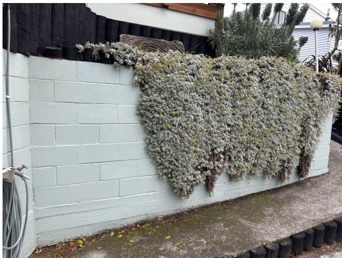
Concrete block walls are showing no evidence of movement or deterioration
