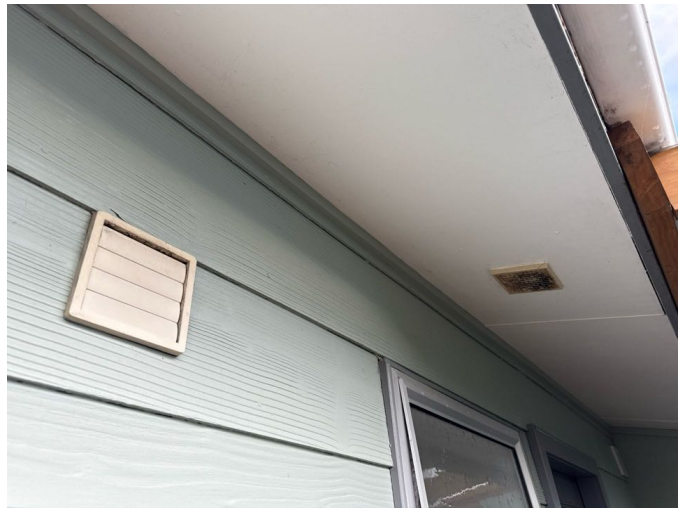
Extraction vents exit through the soffits and walls
