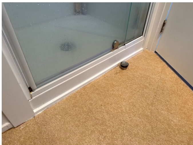
The base of the shower/floor junction appears to be effectively sealed. There is evidence of slight moisture damage beneath. The area must be kept well sealed and moisture managed well to prevent further deterioration.
