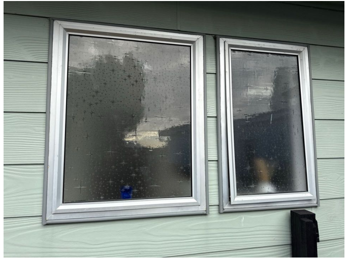
The typical single glazed aluminium window detail consists of a head flashing, timber scribes and sill.
