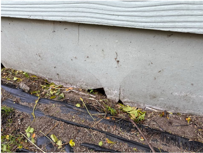
Damage to the base cladding is not a significant concern
