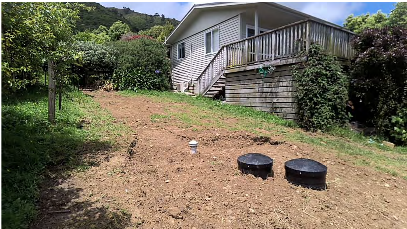
New tank connected from house behind, disposal is to the original field Taken at 1:13 PM on Monday 18/12/2023
