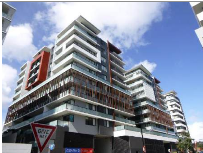
View of southern (front) and western elevations as viewed from the S/W corner area
