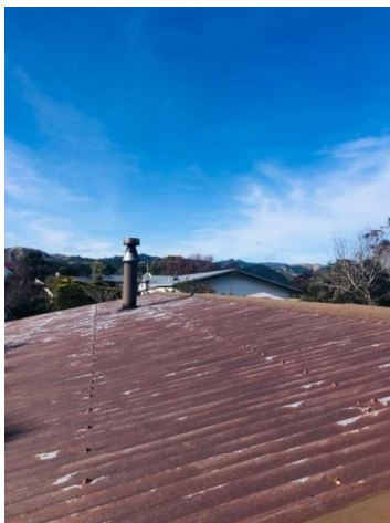
Paint coating flaking.
