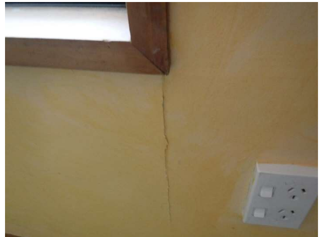
Photo 7. Minor crack observed to the wall lining under the window.
