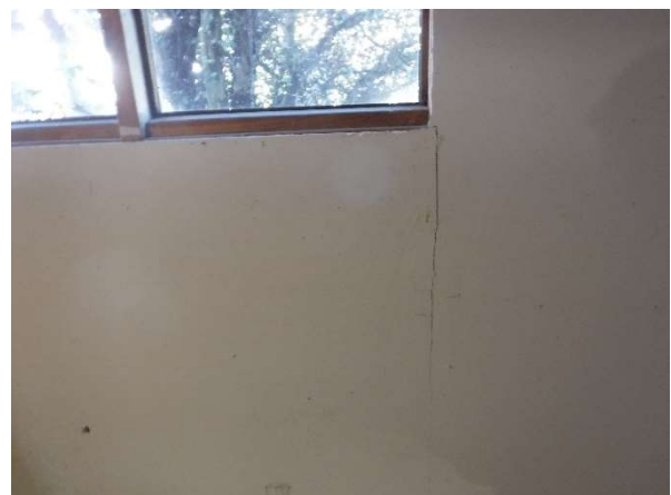
Photo 9. Minor crack observed to the wall lining under the window.
