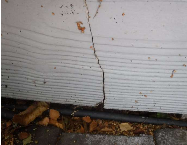
Photo 4. Minor crack observed to the external cladding.
