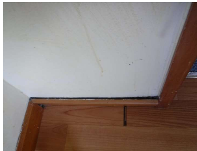
Photo 15. Minor separation observed to the timber skirting.
