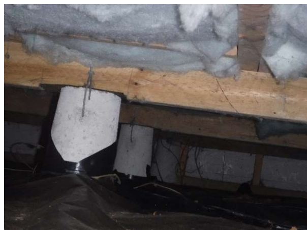
Photo 19. Non-compliant bearer notching observed, there was no splice plates.
