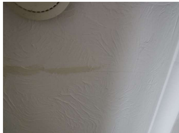
Photo 13. Minor crack and previous repair have been observed to the ceiling.
