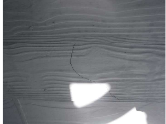
Photo 5. Minor crack observed to the external cladding.
