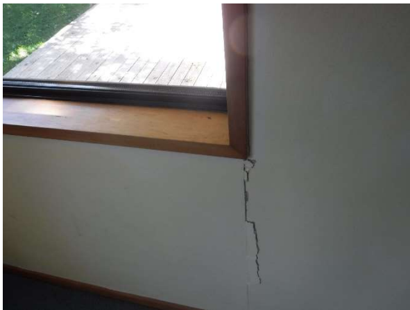
Photo 12. Minor vertical crack observed to the wall lining under the window.
