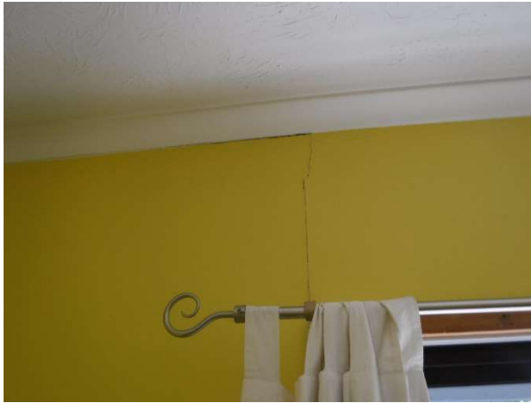
Photo 10. Minor vertical crack observed to the wall lining above the window.
