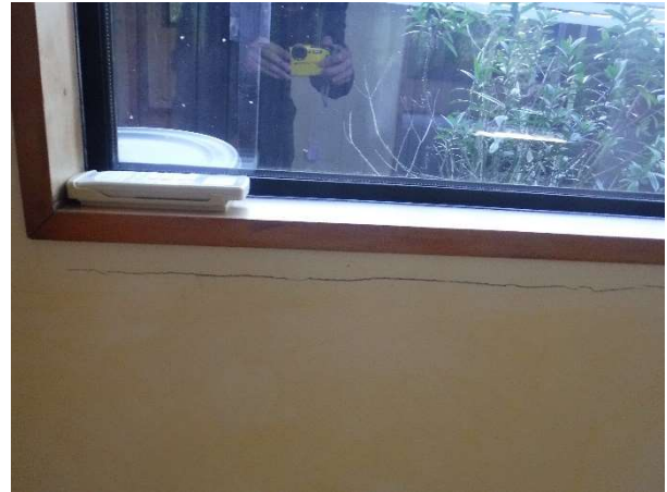
Photo 11. Minor horizontal crack observed to the wall lining under the window.
