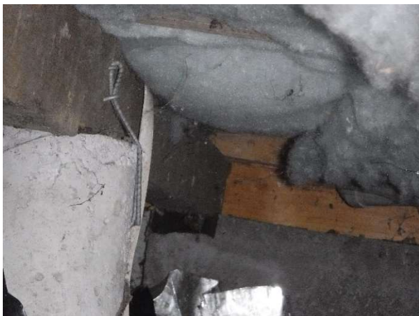
Photo 20. Steel wire connections and no DPC were observed at the pile to bearer interface.
