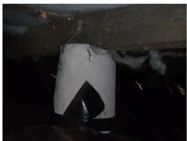
Photo 21. Steel wire connections and no DPC were observed at the pile to bearer interface.
