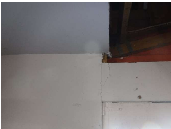
Photo 8. Minor crack observed to the wall lining.
