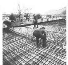
The medules are laid on the pottom layer of steel reinforcement - simply and efficiently.
