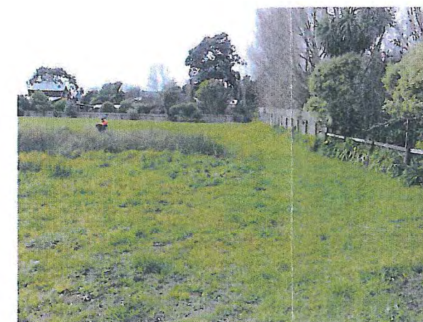
PHOTO 3 EXISTING WETLAND AREA TO BE EXCAVATED TO CLEAN UNDERLYING SAND & FILLED TO RL=5.70
