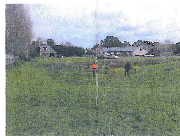
PHOTO 2 EXISTING WETLAND AREA TO BE EXCAVATED TO CLEAN UNDERLYING SAND & FILLED TO RL=5.70
