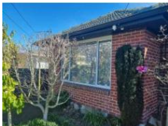
No EQ Mortar cracking noted
