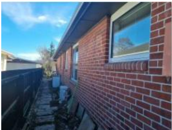
No EQ Mortar cracking noted
