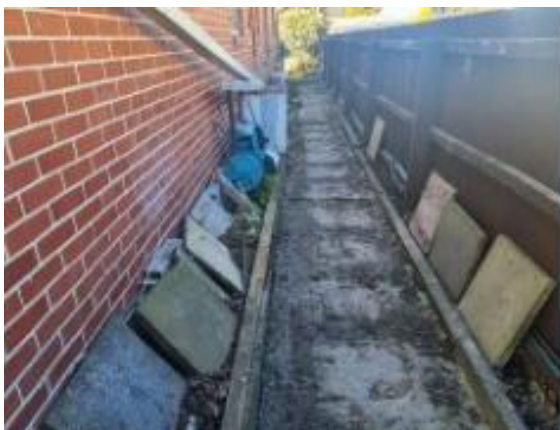
No EQ Mortar cracking noted
