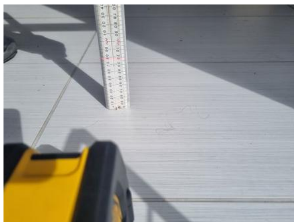
Laser floor level assessment.
