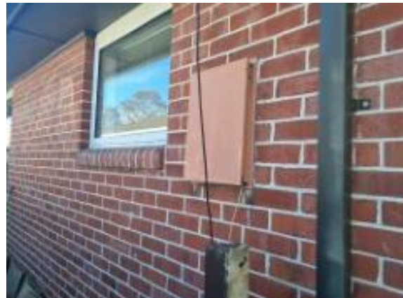
No EQ Mortar cracking noted
