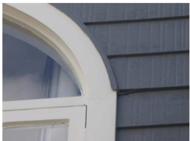
Head flashing detail
