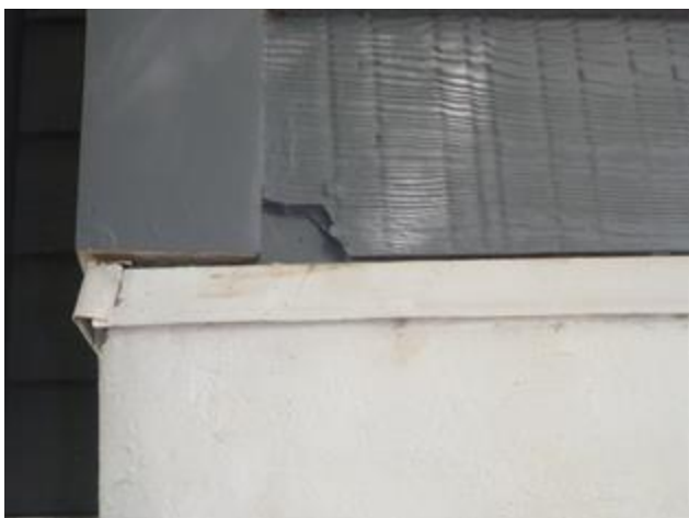
Small area off impact damage
