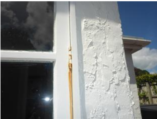
Hinge corrosion
