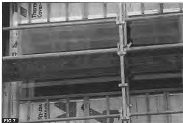
FIG 7 Timber batten cavity with window installed and ALUBAND WINDOW SEALING SYSTEM shown under battens.
