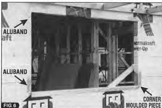
FIG 6 Window opening completed with the Aluband System in place. NOTE: THE ORANGE CORNER MOULDED PIECE AS PART OF THE THERMAKRAFT ALUBAND SEALING SYSTEM.
