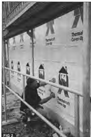
FIG 2 Stud lines are visible for staples, and assists the installer for the placement of staples.
