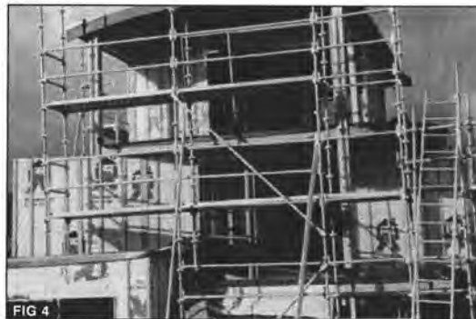
FIG 4 Timber batten cavity over Thermakraft Cover-Up.
