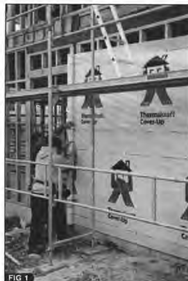
FIG 1 Builders installing Thermakraft Cover-Up . The membrane is kept level by assistance of star lines for stud placements. NOTE: LAP BELOW BOTTOM PLATE.
