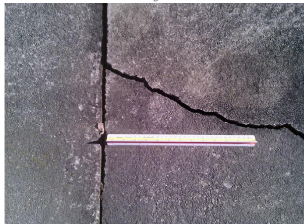
Photo 4: Damage in driveway west of dwelling showing cracks with vertical offset.
