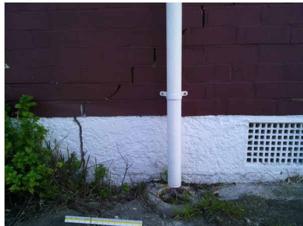
Photo 2: Perimeter and cladding crack in the east side.
