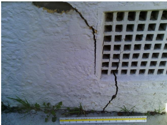
Photo 1: Perimeter crack in the north foundation.
