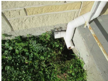
Example of downpipe by deck may need directed to appropriate outlet.
