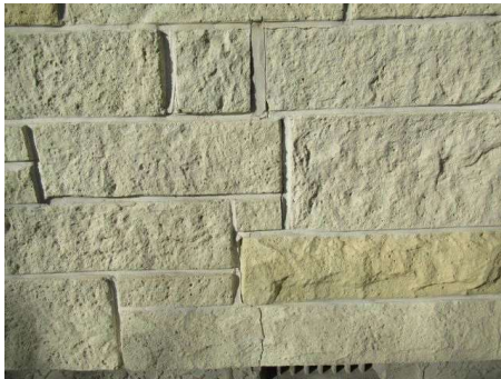
example of step cracking on cladding noted,
