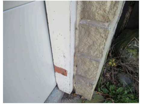
example of borer hole in garage fascia. Treat chemically or replace timber.
