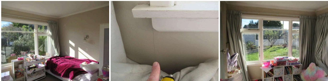
sheet joint movement noted
