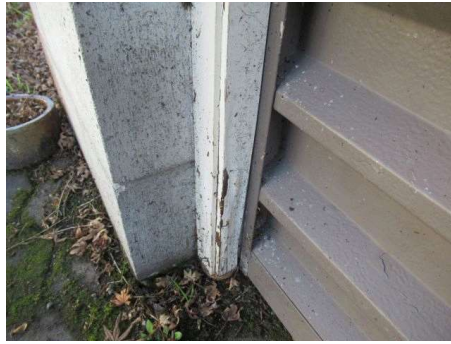
example of soft timber fascia on small garage door, repair/replace noted
