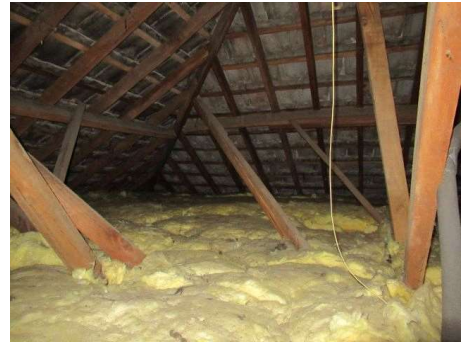
Ceiling insulation in generally good condition, unable to sight all
