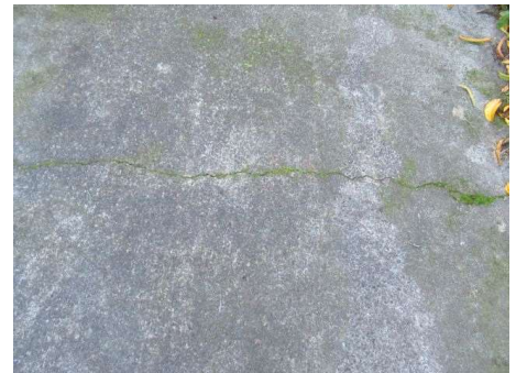
example of cracking in paths, noted, appears sound
