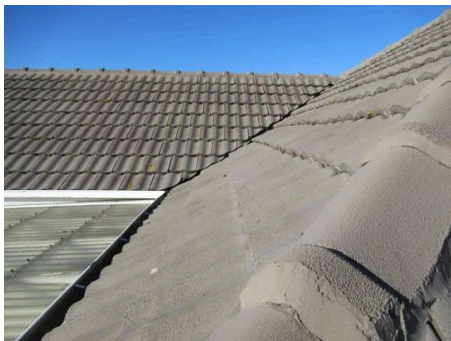
hip tile may need repositioning noted.
