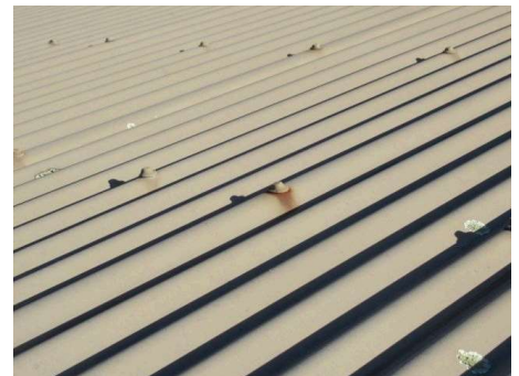
example of garage roof surface rust/ clean/prime to prolong life, check fixings
