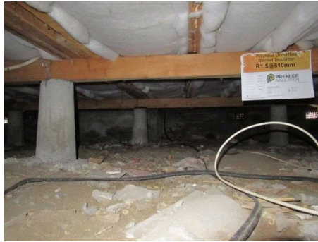
sub floor, and insulation is in generally good condition, unable to sight all
