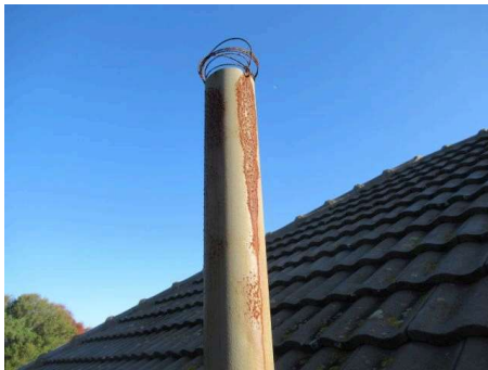
example of surface rust on roof vent pipe, clean/treat and paint to extend life.
