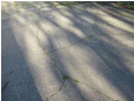
example of cracking in driveway noted
