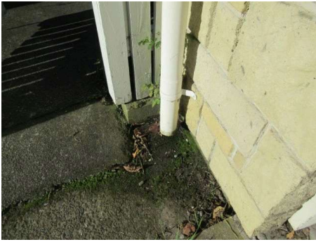
Downpipe at on garage needs directed to a stormwater outlet,
