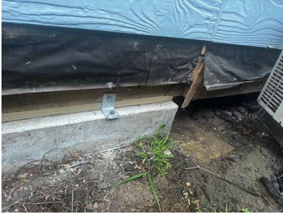
Photo 1. Over-pinning connection detail observed.
