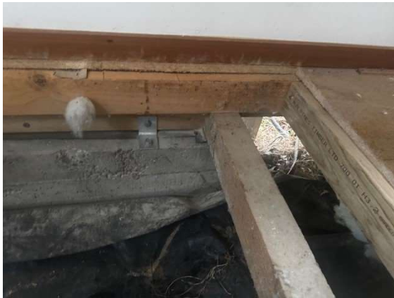
Photo 5. Steel bracket observed for the over-pinning connection detail.
