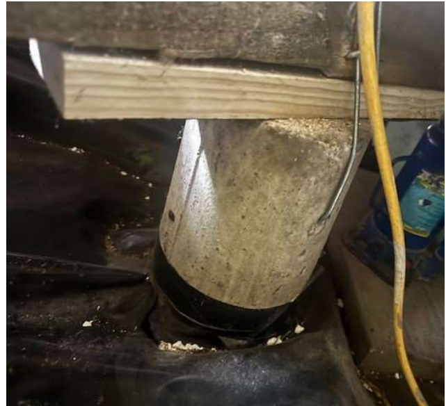
Photo 4. Internal pile packing detail observed.
