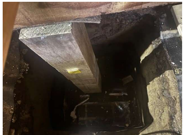
Photo 8. Pile hole for new timber pile observed.
