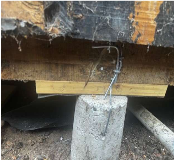
Photo 3. Internal pile packing detail observed.
