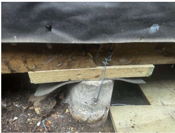
Photo 7. Internal pile packing detail observed.
