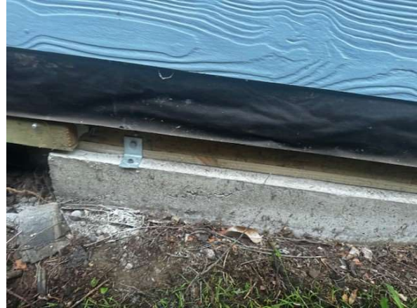
Photo 2. Over-pinning connection detail observed.
