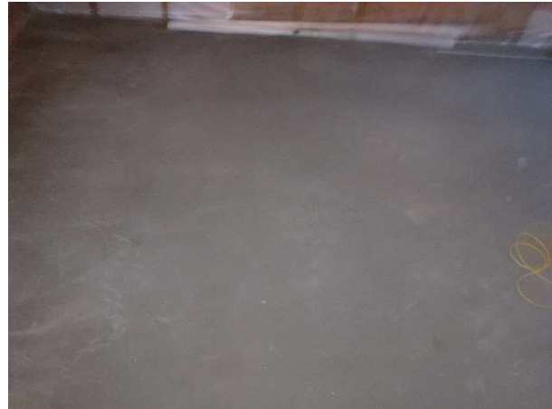
Photo 14. Sika Floor Levelling Compounds applied.
