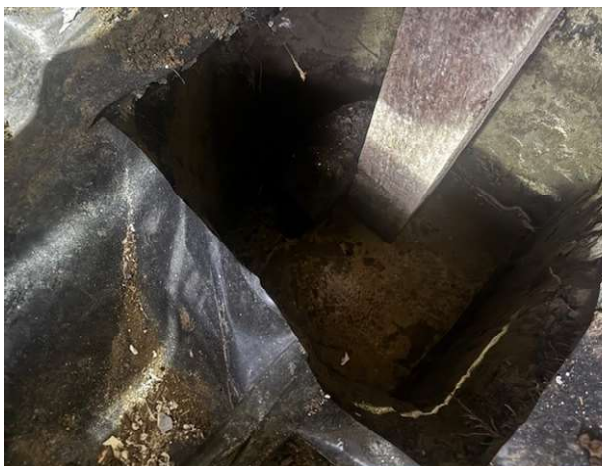
Photo 9. Pile hole for new timber pile observed.
