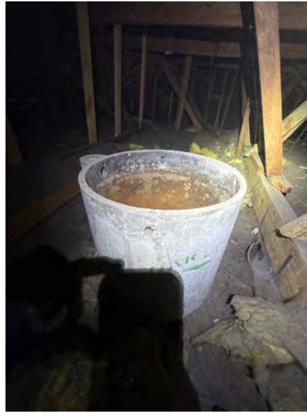
Remove obsolete header tank from the ceiling cavity.
