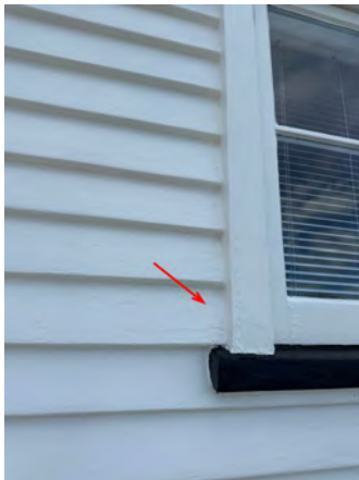
Some rotting under paintwork here.
