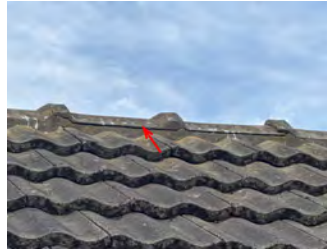
Example - typical cracking and separating to mortar on tile capping in places.
