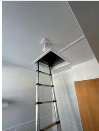
Ceiling cavity access in the laundry.
