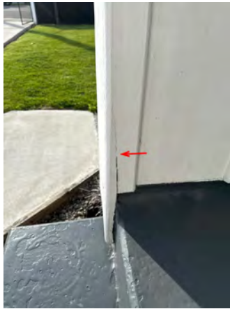
Cracked batten.
