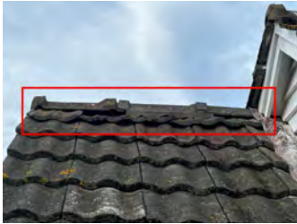
Crumbling mortar needs filling and tiles re-fit so they don't sit up.
