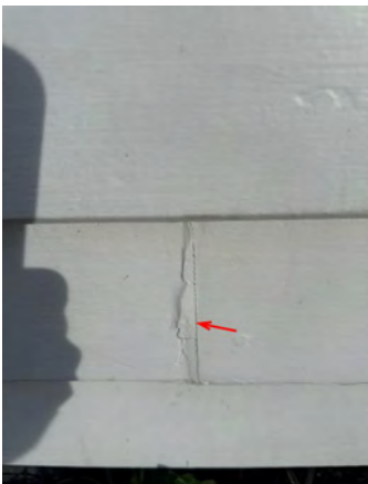
Example - check over and gap fill any weatherboard joins that have re-cracked. This will help protect the boards from moisture intrusion.
