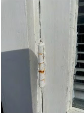
Example - typical rusting to some hinges. Some window hinges have been replaced.
