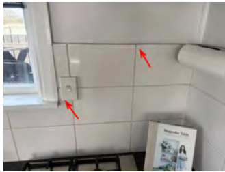
Movement in tiles and cracking to grout.
