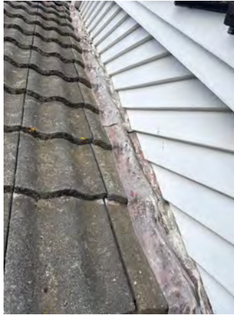
Crumbling mortar needs filling and tiles re-fit so they don't sit up.
