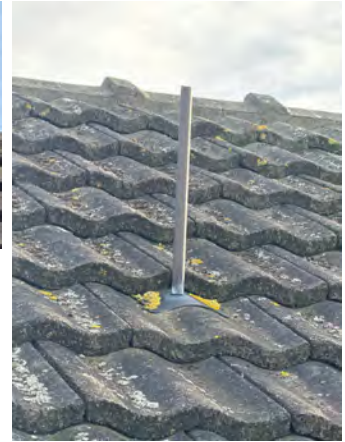
Example - typical cracking and separating to mortar on tile capping in places.
