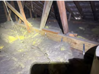
Retrofit beam where load bearing wall has been removed. Looks to have been professionally done.
