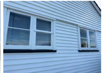
A lot of filler has been used on these western window frames. This indicates previous or current rot.
