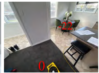
Heights adjusted for floor coverings.
