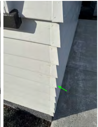
Metal corner soakers have been fitted to some corners. These help protect the weatherboard ends from moisture damage.
