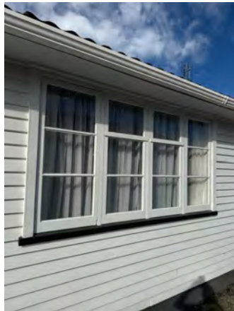
A lot of filler has been used on these western window frames. This indicates previous or current rot.
