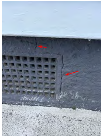
Example - some typical movement cracking around some sub floor vents.
