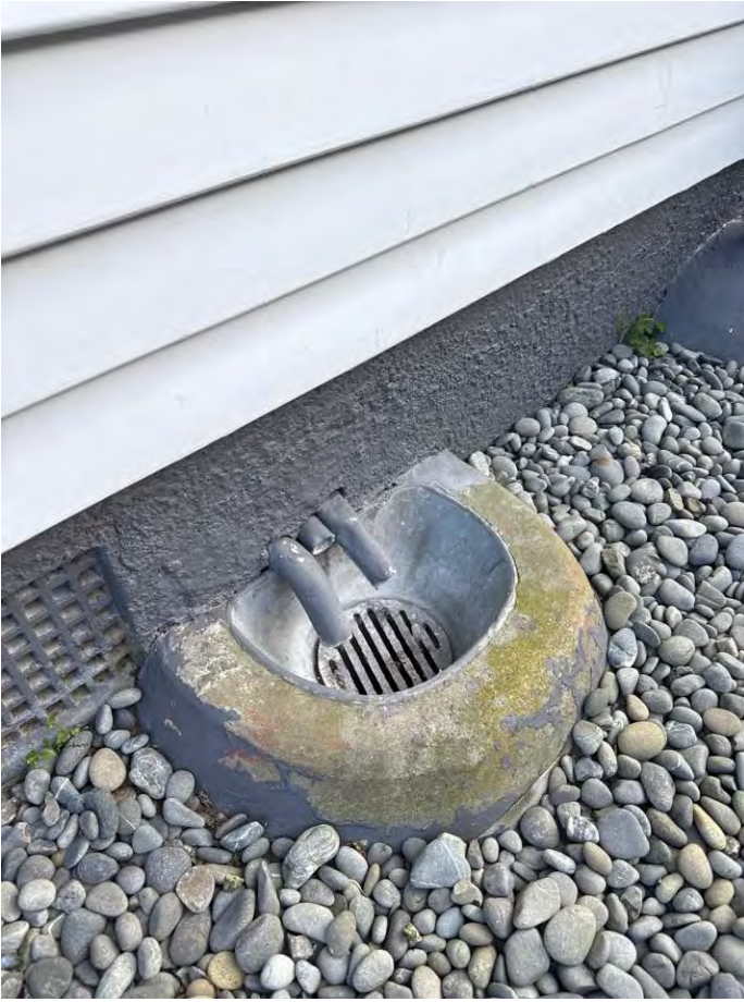
These gully trap pipes are above the grate and could be extended below the grate.
