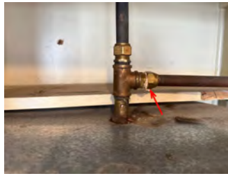
Corrosion to fitting.
