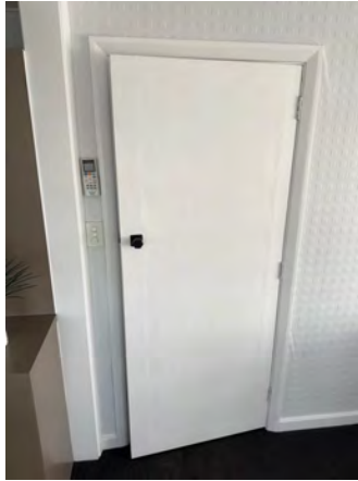
Adjust striker plate so door latches.
