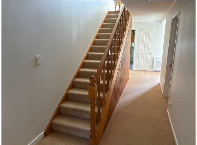
The timber stairs and balustrade are solid and secure
