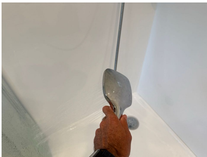
Good water pressure noted. No sign of current leaks from the shower frame during water testing.
