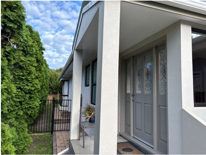
Roof supports are solid and secure
