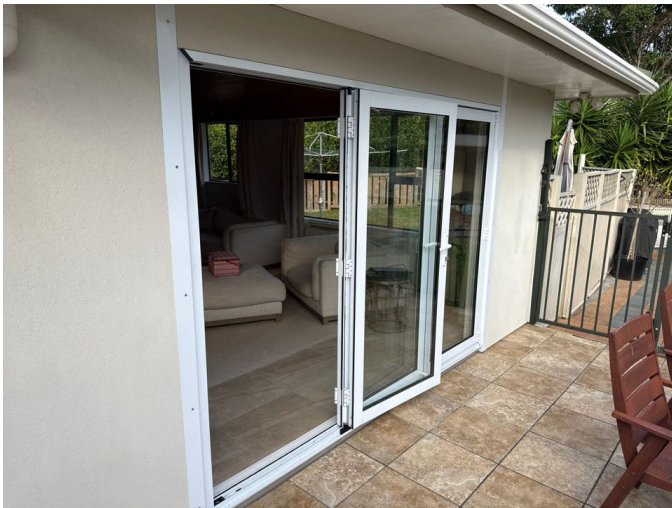
A double glazed aluminium bifold door unit has been installed by the patio. The unit appears to be effectively flashed and is in good condition.
