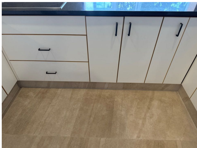
The kitchen cabinetry and tile floor are in good condition
