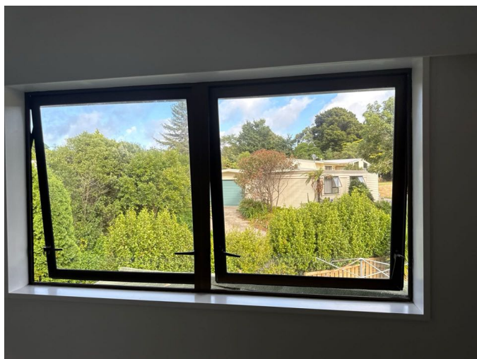
The windows are functioning throughout
