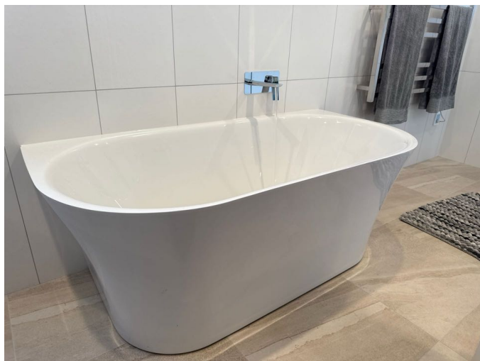
The back of the bath is well sealed. The tap is functioning well.
