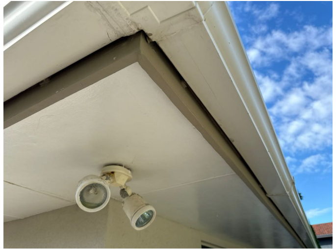
Average paint quality to the timber fascia, barge boards and fibre cement soffit linings
