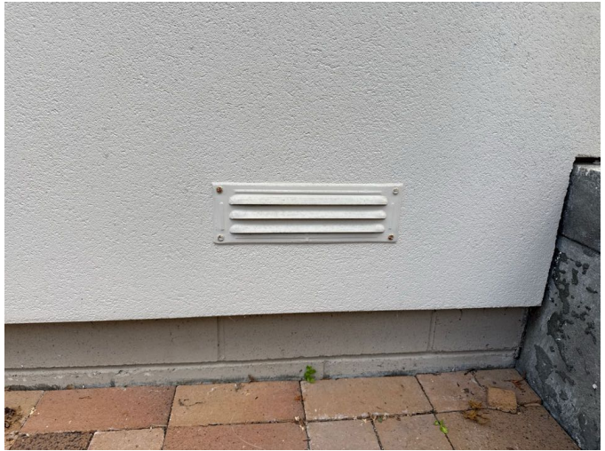
Sub floor vents installed in some areas
