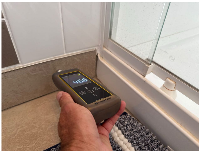
The common fail areas of the shower were checked for elevated moisture. Moisture levels were within the normal range.
