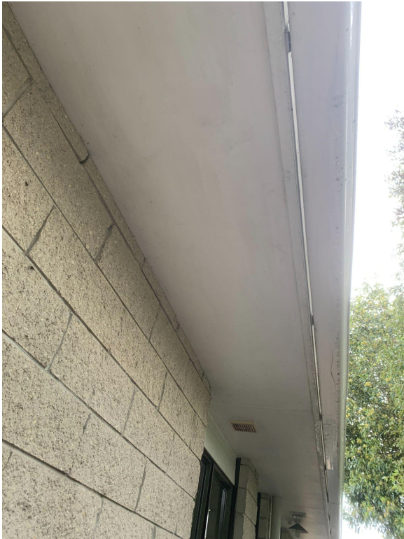
Photo 12: Ends of barge boards sanded and repainted.
