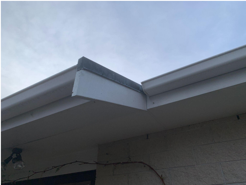
Photo 12: Ends of barge boards sanded and repainted.
