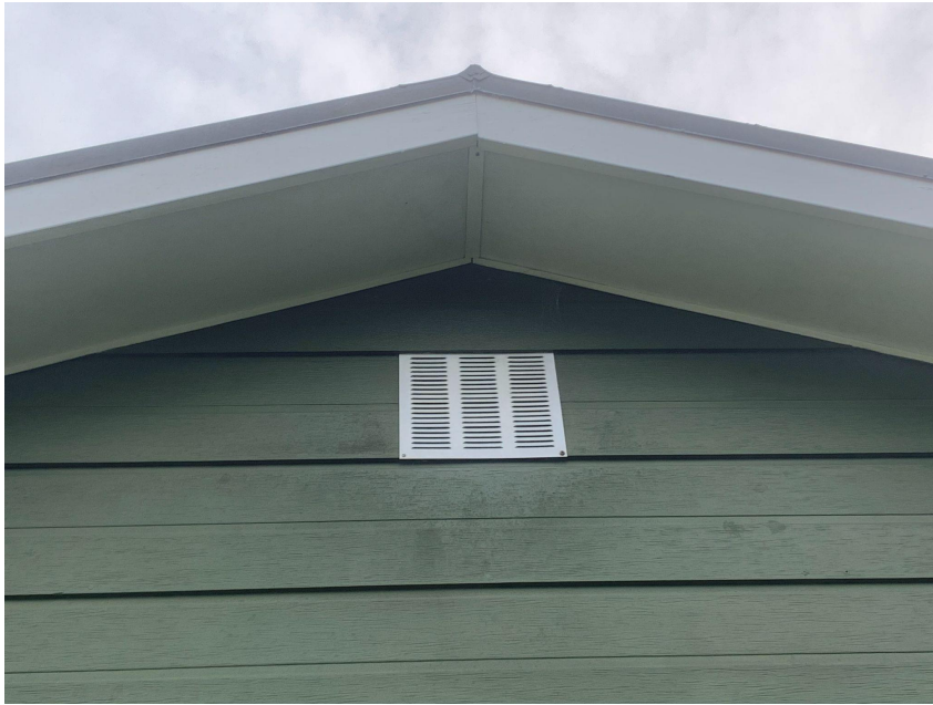
Photo 13: Fascia sanded and repainted, jointer capping replaced.
