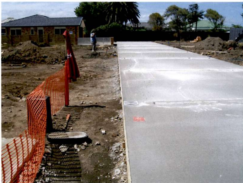
New ROW with swale and soak holes
