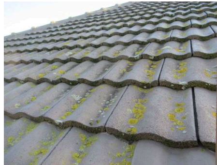
example of lichen on roof ,treat chemically to control
