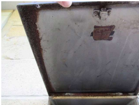
example of surface rust on meter box cover noted, clean/ prime and paint
