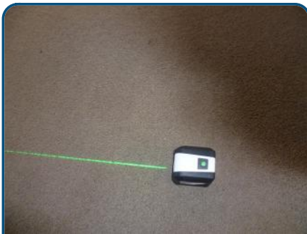
Laser floor tec used, green laser should be 45mm above floor
