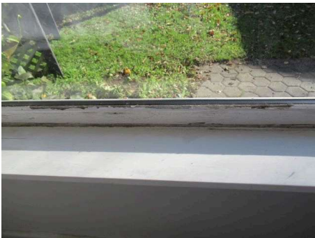
surface wear to window timber paint, can repaint noted noted,
