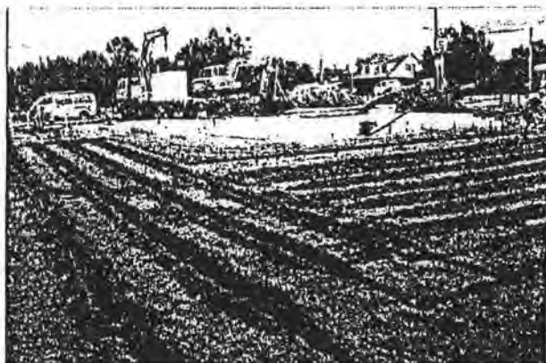
Installing drip irrigation lines into existing lawns causes little disruption and can be completed before your house is built.
