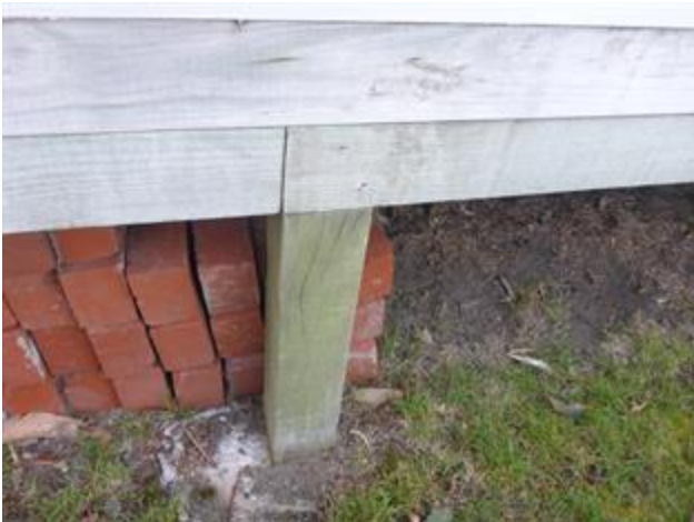
Additional support to bearer join
