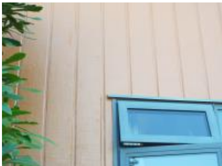
good flashing detail
