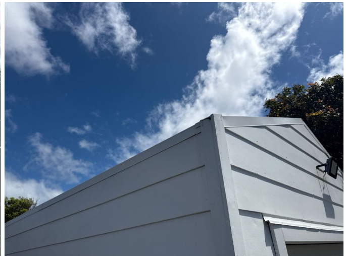
There are no barge boards or fascia under the barge flashings. This is a high weather tightness risk.
