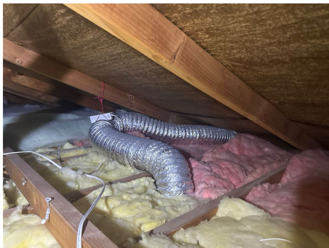
Extraction units vent to the exterior
