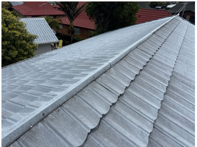
The roof flashings appear to be secure, intact and are effective. No sign of failure could be found beneath where accessible to view.
