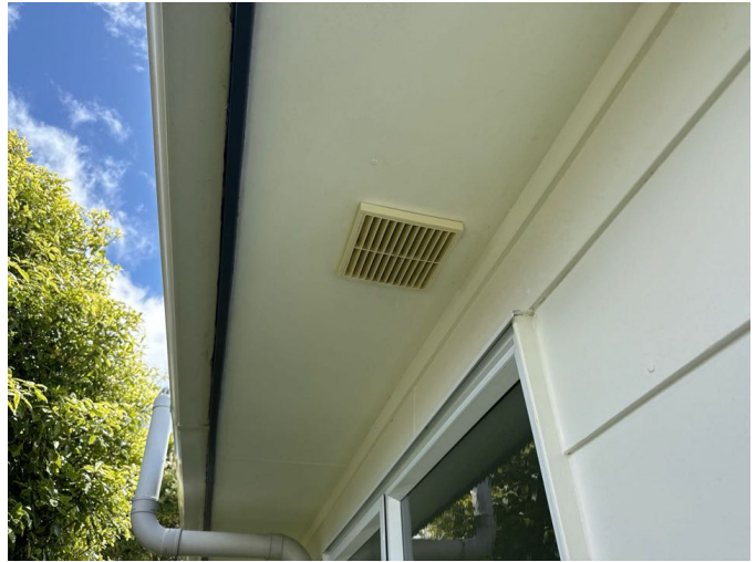
Extraction vents exit through the soffits
