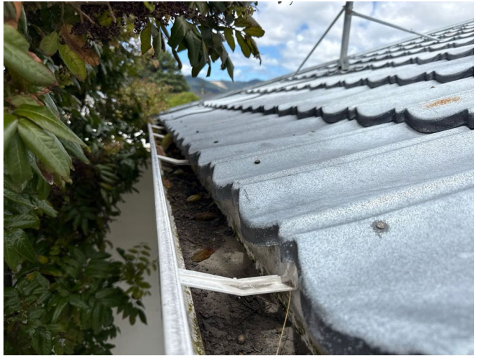
The spouting is in need of a clean out which will help prevent the risk of blockages and overflows. The effectiveness of the spouting will need to be checked during rainy periods. Due to the dry conditions that were evident on the day of our inspection we cannot comment on any leaks that maybe evident to the spouting or down pipes.
