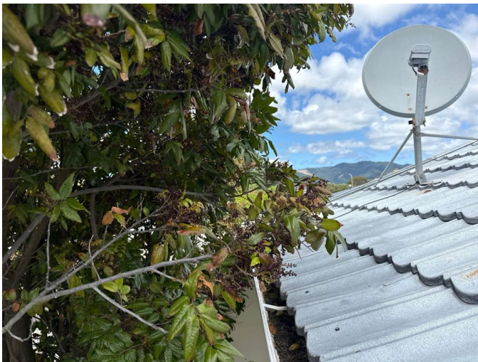
Trees overhanging the roof should be trimmed back to prevent the risk of blockages to the spouting.
