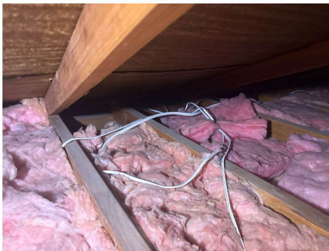
Only modern TPS wiring sighted during the inspection which is consistent for the age
