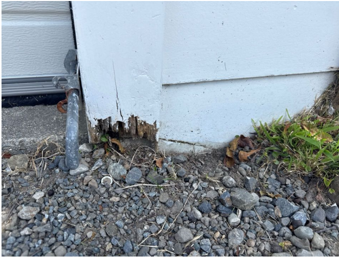
Damage to the timber facings and bottom weatherboard. Replacement recommended.
