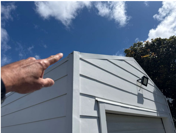
The corner facings have been poor detailed and are a weather tightness risk at the top. A licensed builder should be engaged to improve this detail.
