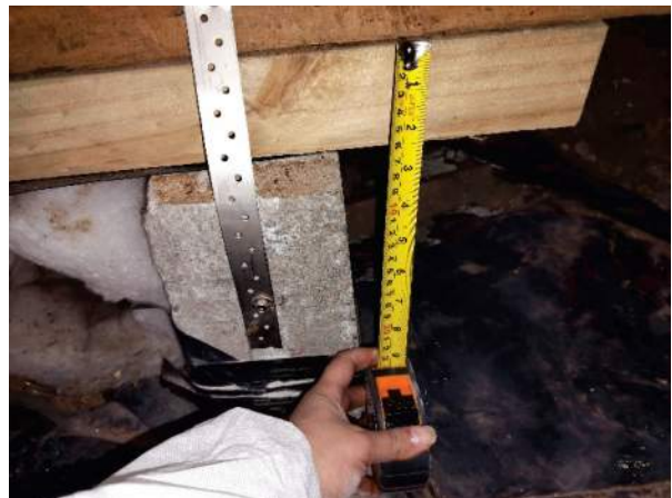
Photo 4. View of the existing concrete pile, sub-floor connection, and packer (2).
