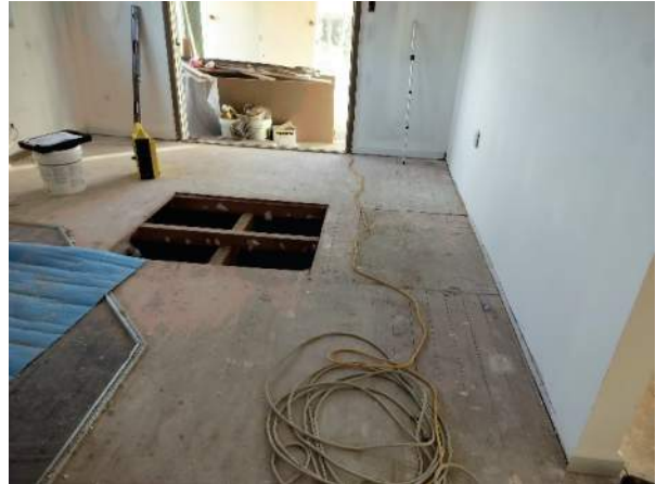
Photo 2. View of the re-levelled (lowered) floor by bearer notching method.
