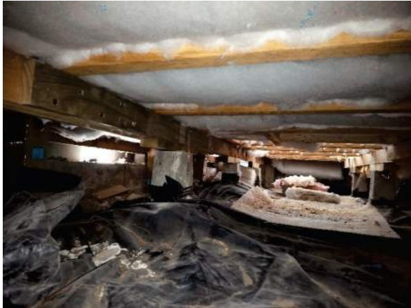
Photo 1. View of the re-levelled (raised) floor by mechanical lifting method.
