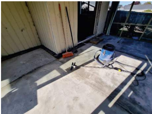
Photo 3. View of the re-levelled (raised) floor by FLC method.
