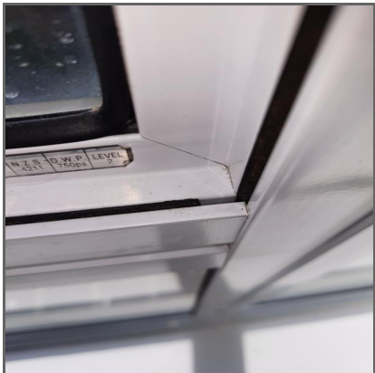
Weather seals are incomplete and not effectively sealing the window.
