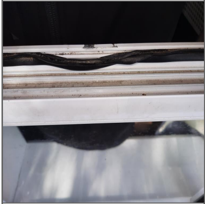
Weather seal is damaged and will need to be replaced.
