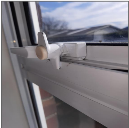
Window handle on the right hand side is missing the catch tongue and not effectively holding the window shut.
