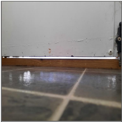
Large gap under the door where cold air can be felt passing through.
