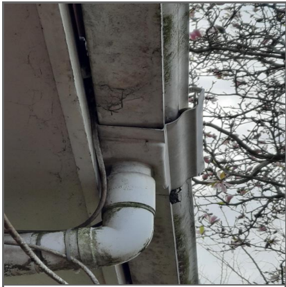
Gutter on the left hand side of the property is disconnected and damaged.
