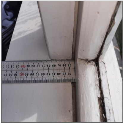
2 x window casements have large gaps and will need to be eased so they close tightly against installed weather seals
