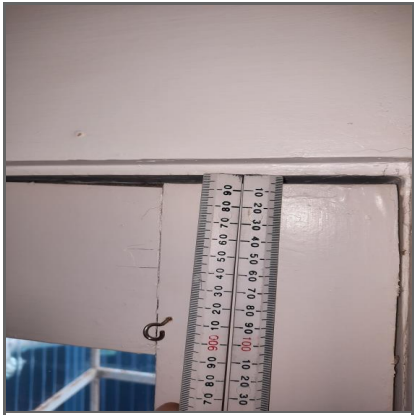
5mm gap at the top of the door where cold air can be felt passing through.
