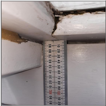
Bottom right hand casement has non effective existing weather seal and 7mm gap at the bottom. Air can be felt passing through.
