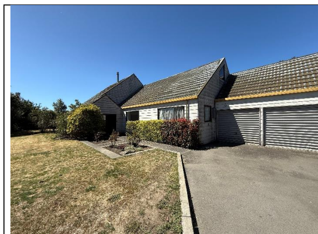
Southwest elevation (front)
