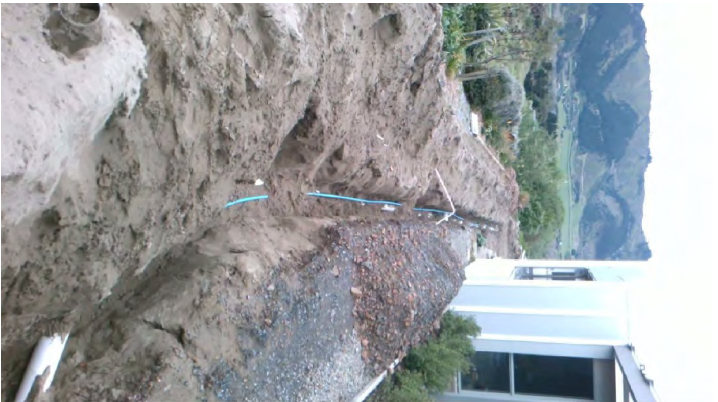
New drain run to addition apprx 20M Taken at 12:10 PM on Wednesday 12/06/2019
