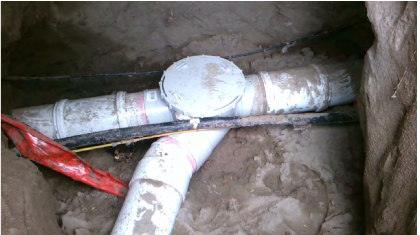
connection to existing immediately prior to septic system Taken at 12:09 PM on Wednesday 12/06/2019
