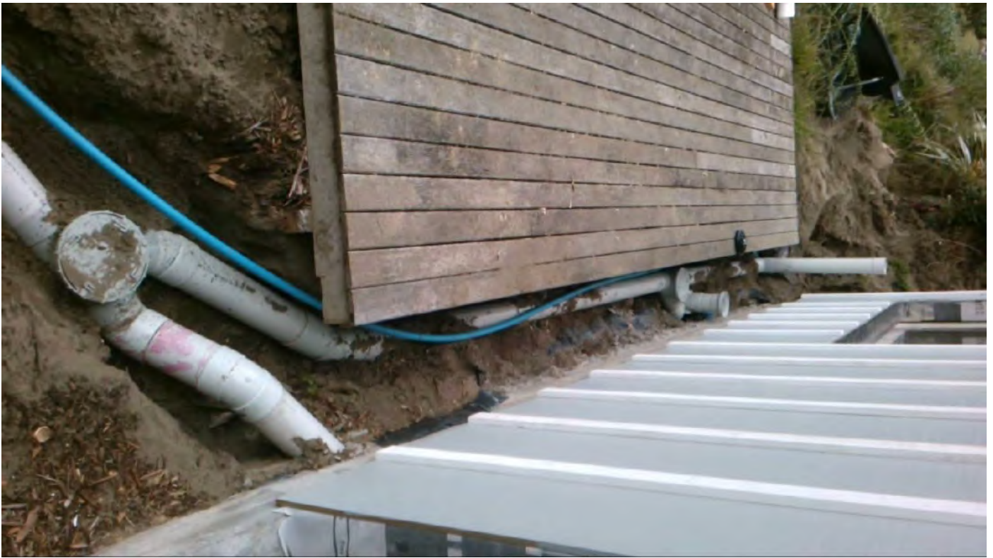
ORG charged, vent at end of line, requires to be downstream of fixture Taken at 12:11 PM on Wednesday 12/06/2019
