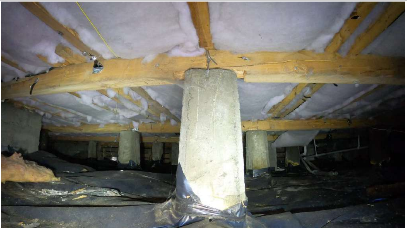
36: Here we see that the bearer has been notched and not reinforced. The bearer has also cracked. We can't see it here but in shot 48 of the other side of this pile we see that it is cracked.
