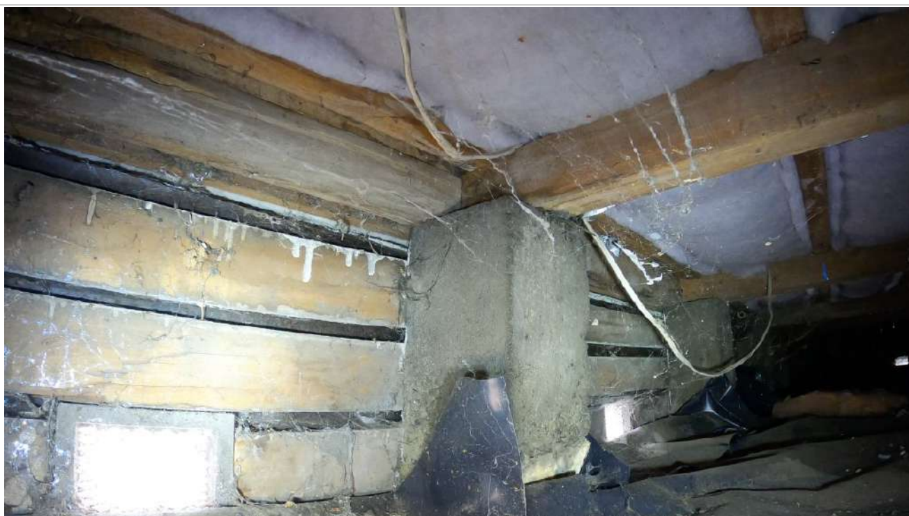
32: Cast in place concrete pile.
