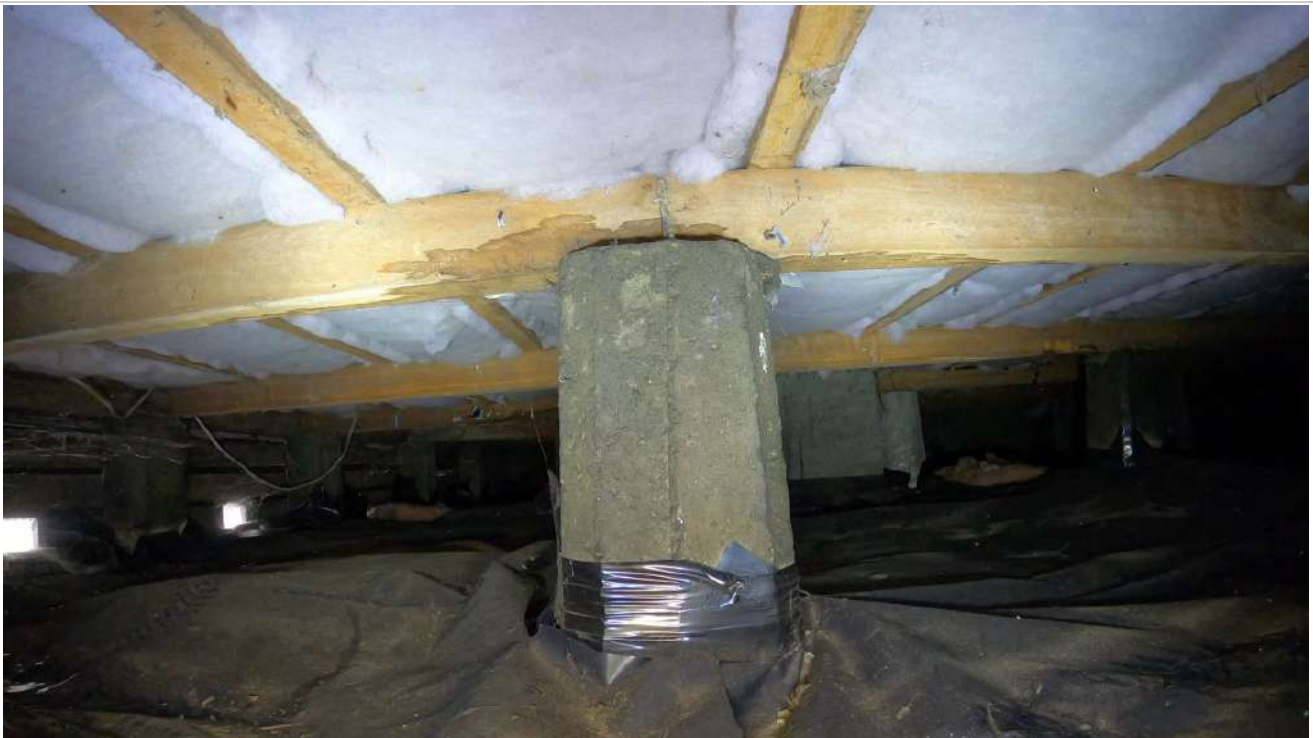
18: The home has precast concrete piles. These maybe concreted into the ground but the polythene obscures this. They are connected to the bearers with stapled off wire ties. We do see a couple of broken ones.
