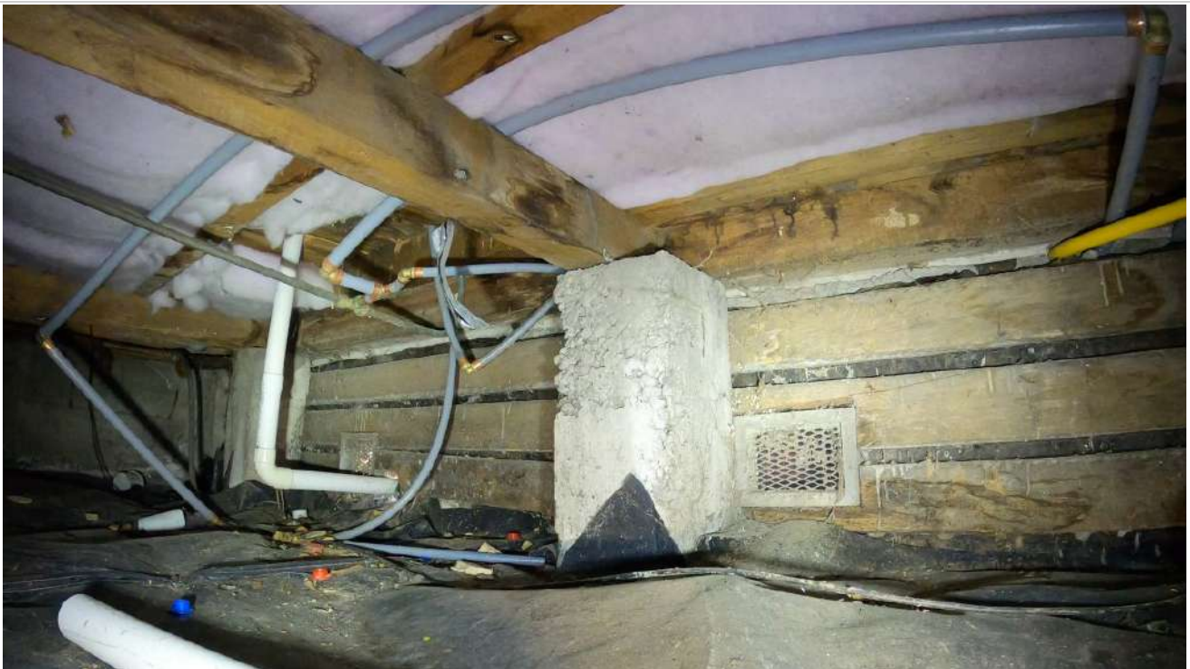
40: Cast in place concrete pile. There has been a water leak in this area which may have been fixed but the timber has been damaged.
