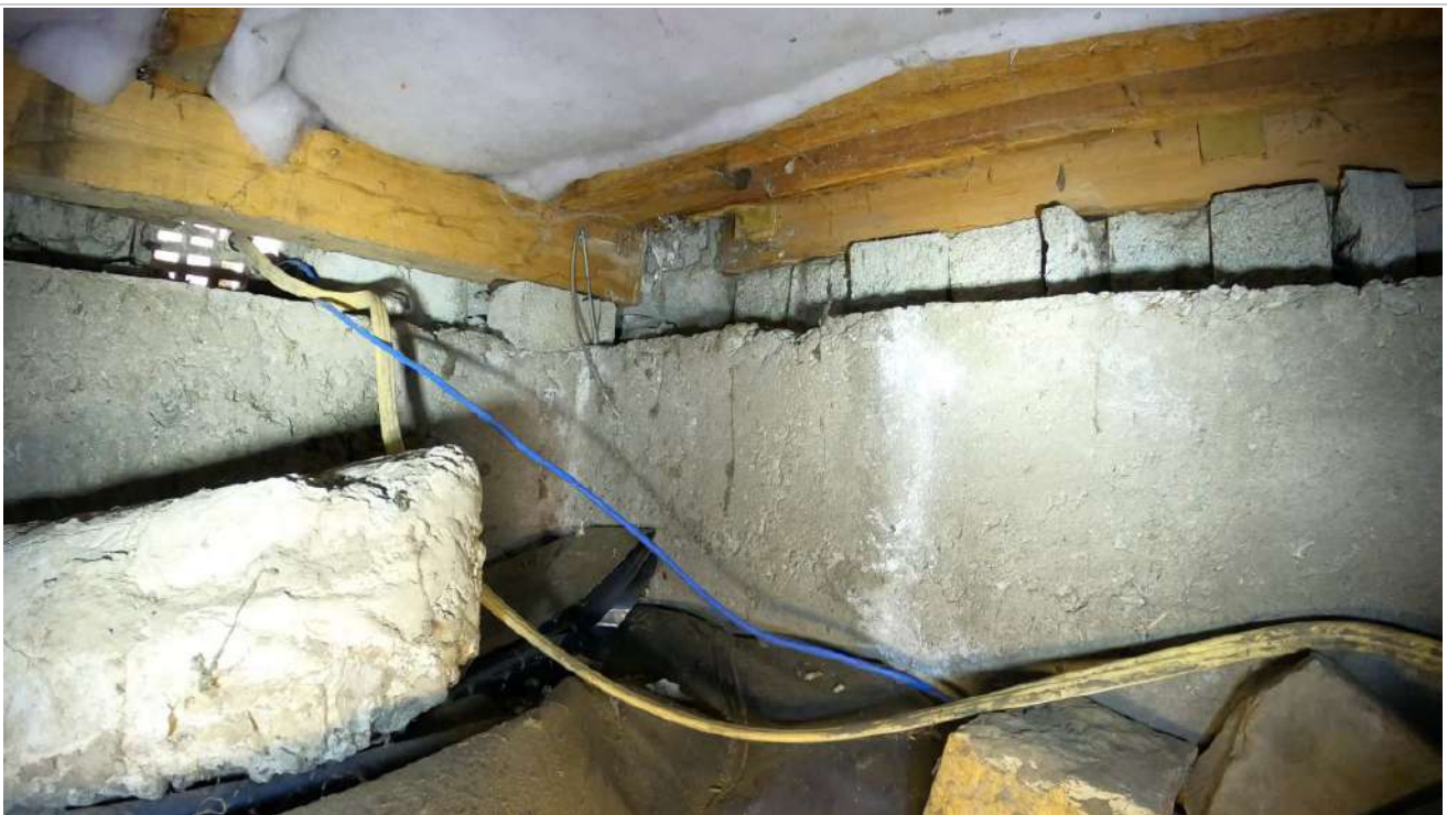
8: View of ring foundation. There are some non-compliant issues with the wiring seen in this home. They could also be a significant hazard to anybody operating under the floor. This relates specifically to unclipped wires. An electrical inspector could be consulted regarding this. The communication cable has also not been laid in a compliant manner and would easily be damaged by people accessing the subfloor.
