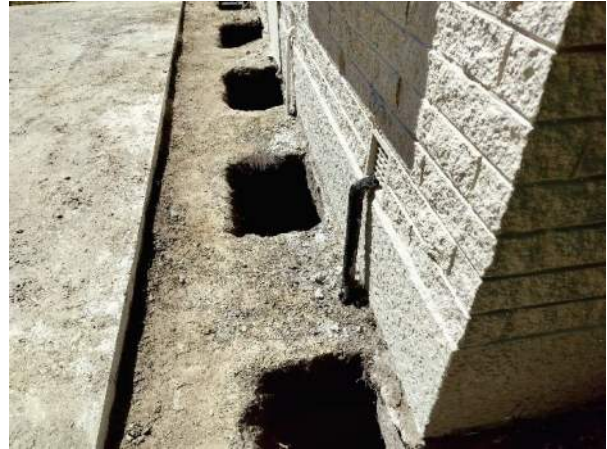
Photo 2. View of excavated pits for underpinning pads (1).
