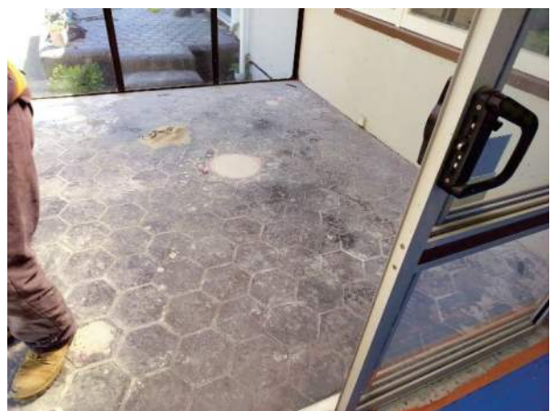
Photo 12. View of internal slab floor in Sunroom post re-levelling .
