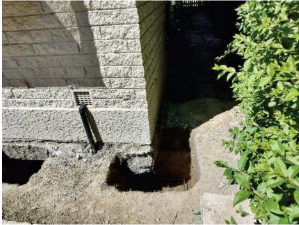
Photo 1. View of excavated pits for underpinning pads.
