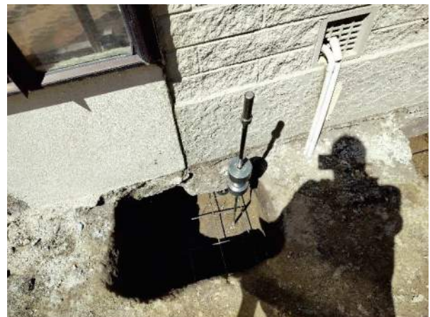
Photo 6. View of excavated pit for underpinning pads (5).
