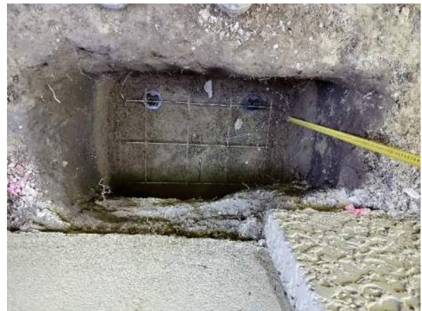
Photo 4. View of excavated pits for underpinning pads (3).
