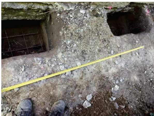
Photo 5. View of excavated pit for underpinning pads (4).
