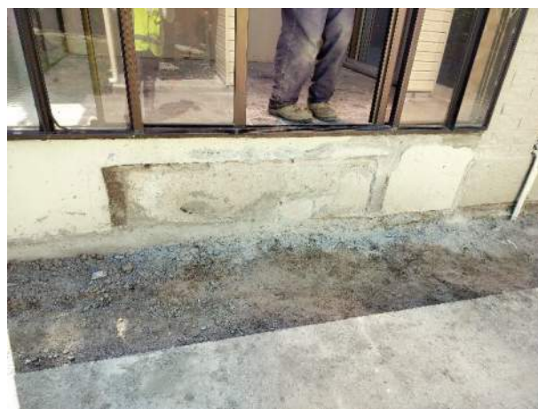
Photo 11. View of crack repaired to the perimeter foundation.
