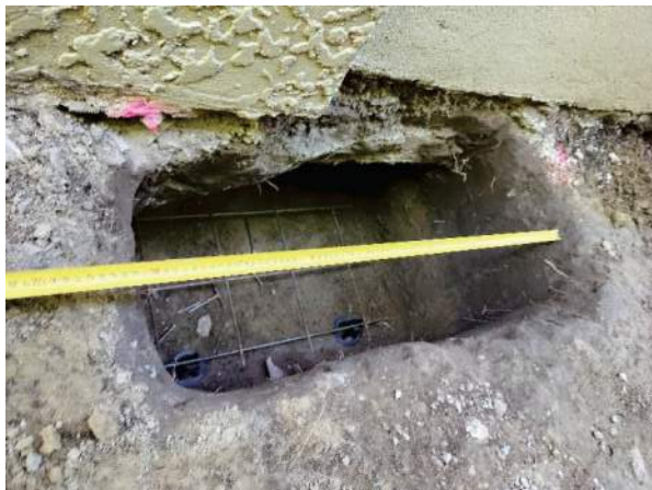
Photo 3. View of excavated pits for underpinning pads (2).
