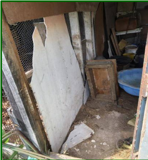
Photo 7 – Large shed with ACM material
