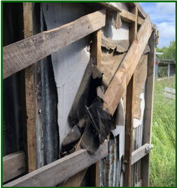
Photo 8 - Shed door with ACM lining.
