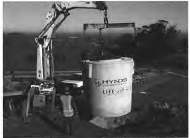
Figure 13: Installation of a Lifestyle system
