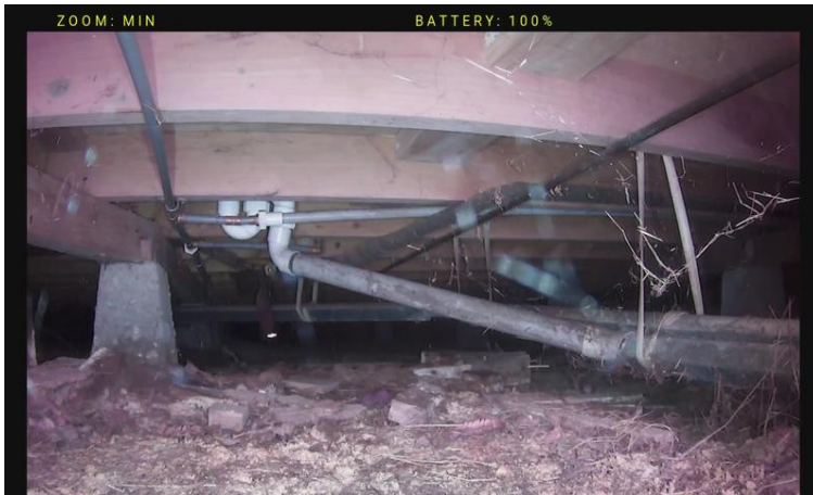
Photo 14 Water and waste pipes are supported.
