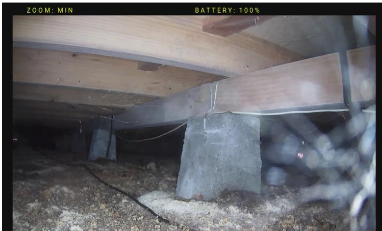
Photo 16 Pile and bearer connections are visible.
