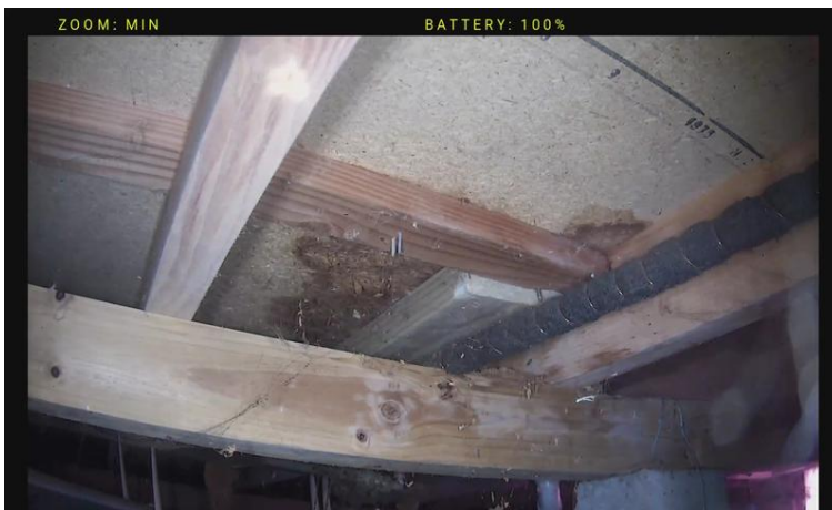
Photo 15 Moisture stains visible under the bathroom/toilet area.
