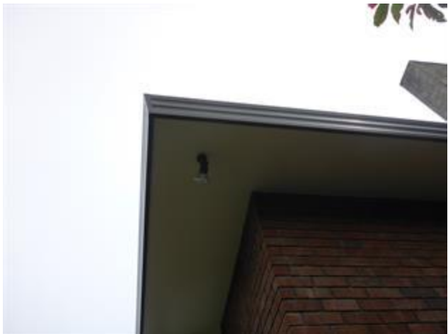
Cement board soffits/metal fascia
