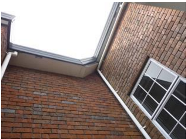
Cement board soffits/metal fascia
