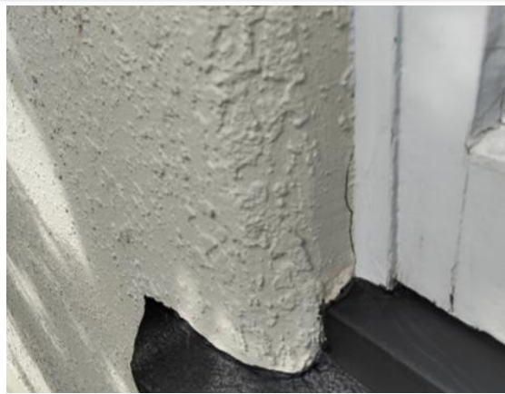
Small crack in the plaster adjacent to the window on the front elevation of the dwelling
