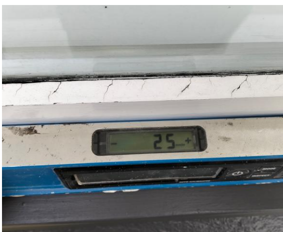
Windows and doors are out of level and/or plumb
