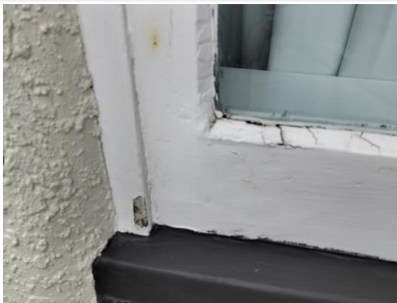
Some paint maintenance required on the timber windows
