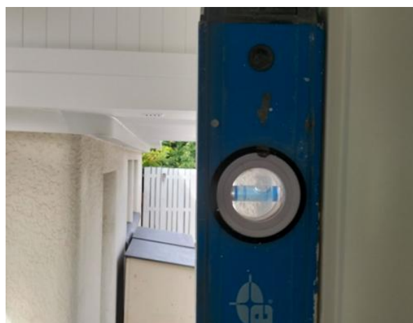
Windows and doors are out of level and/or plumb
