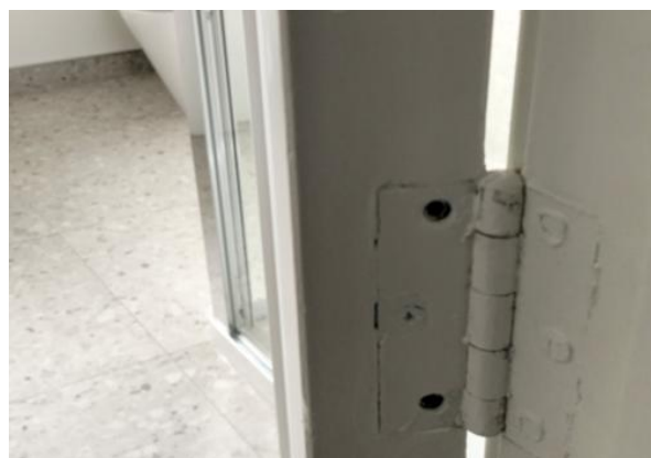
The bathroom door hinges are missing several screws
