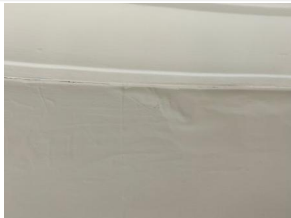
Loose plaster just below the cornice in the bedroom at the end of the hallway
