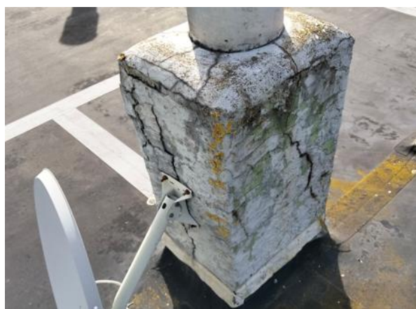
Plaster on the chimney is cracked/broken
