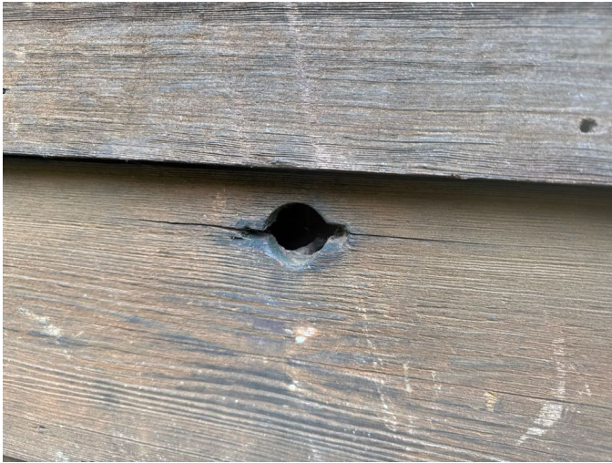
The hole in the cladding should be waterproofed
