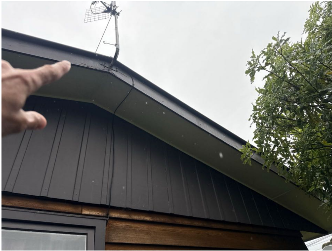
Paint deterioration to the timber barge boards
