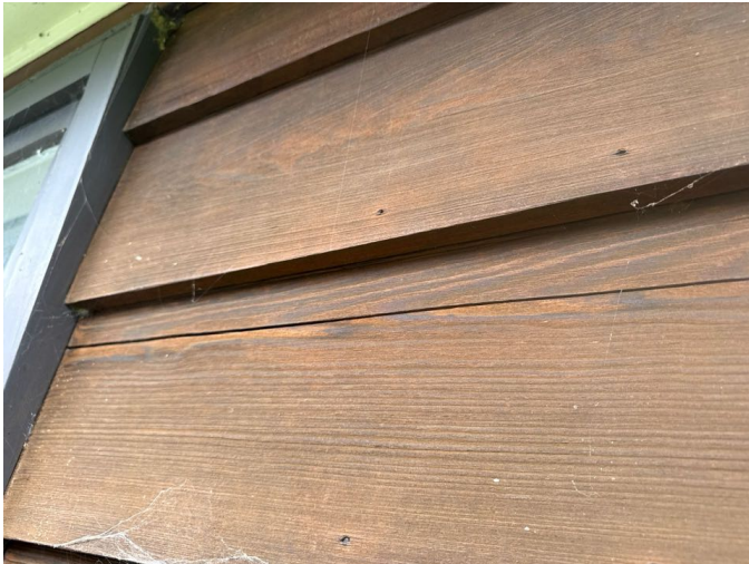
Example. Any cracks such as this should be thoroughly sealed or the boards replaced.
