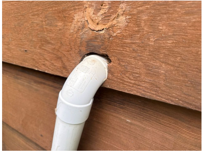
Cladding penetrations in general are a weather tightness risk area. Penetrations such as taps, screw fixings, gas or water pipes etc. A good seal must be maintained around all cladding penetrations over time to prevent issues. No evidence of failure could be found however any gaps should be sealed.
