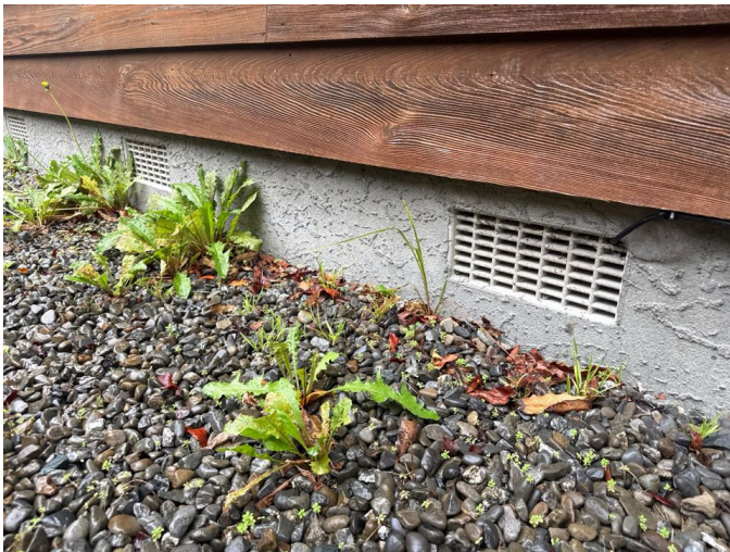
Good ground clearance around the perimeter. The current building code requires a 150mm clearance between the internal floor height and the sealed ground and 225mm to unsealed ground.
