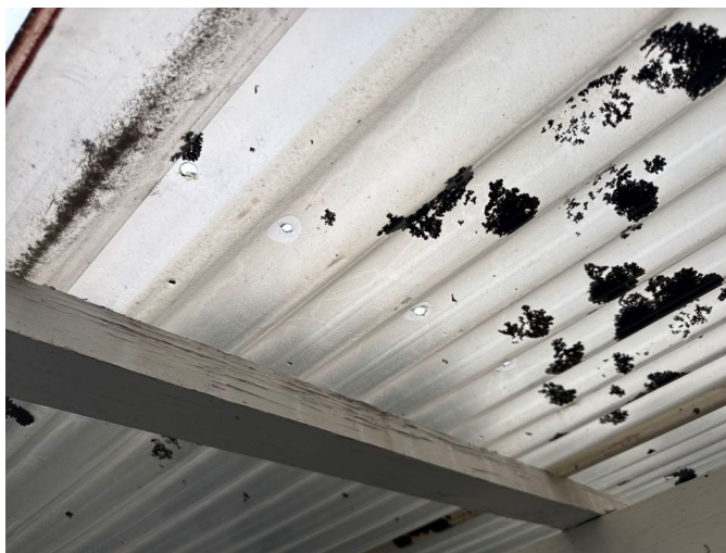
The plastic carport roof has holes from old fixing points
