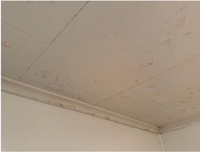
Paint deterioration to various locations
