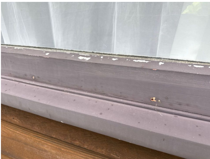
The timber windows and doors require a paint upgrade where surface wear is present.
