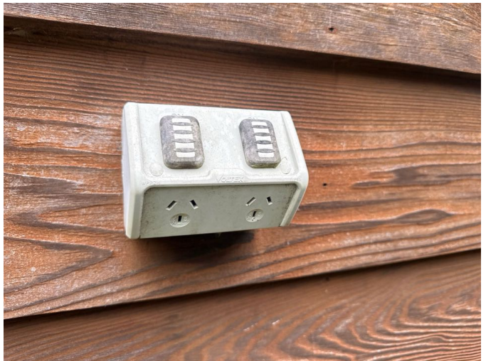
External power point noted. Untested.
