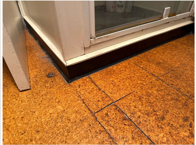
The flooring is deteriorating and should be replaced to prevent the risk of damage to the floor beneath
