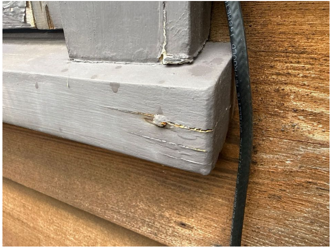
Rust affected nails need to be treated with rust converter and painted
