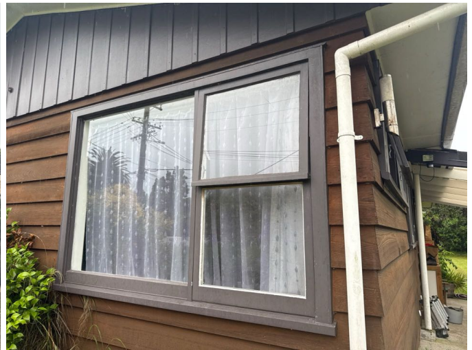
The typical single glazed timber window detail consists of a head flashing, timber scribes and sill.
