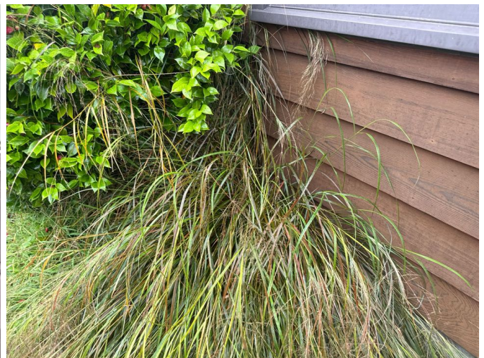
Plants in close contact with the cladding should be trimmed back to prevent the risk of premature deterioration
