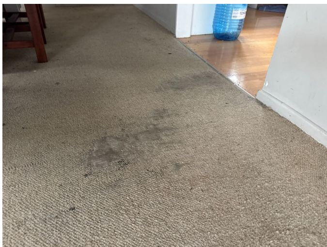
The carpet is very worn and is due for replacement
