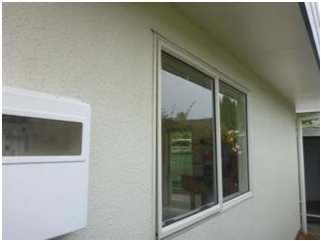
Metal head flashings fitted
