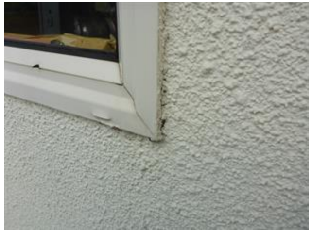
Poor seals to the joinery/cladding junction
