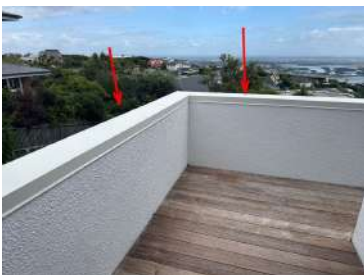
Parapet flashings
