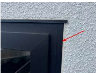
Window silicon seals
