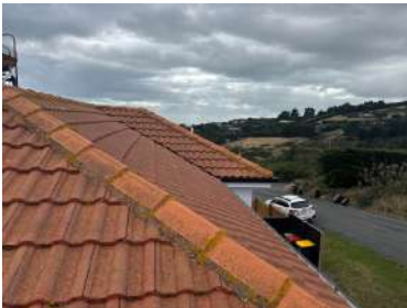
Concrete tile roof with hip and ridge cappings
