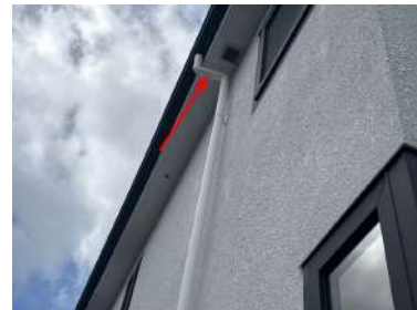
All downpipes connected to the gutter correctly
