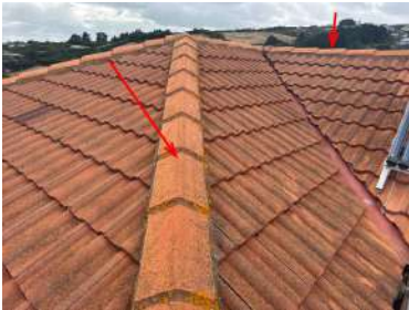
Concrete tile roof with hip and ridge cappings
