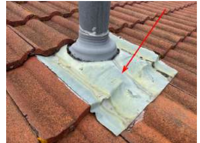
Chimney penetration flashing
