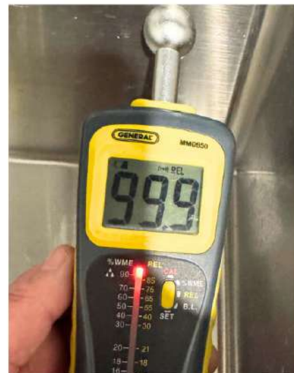
High moisture reading: Red: Damp = 20+ Wet = 50+
