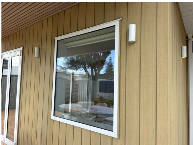
The typical double glazed aluminium window is face fitted with a head flashing and timber bead at the sides.
