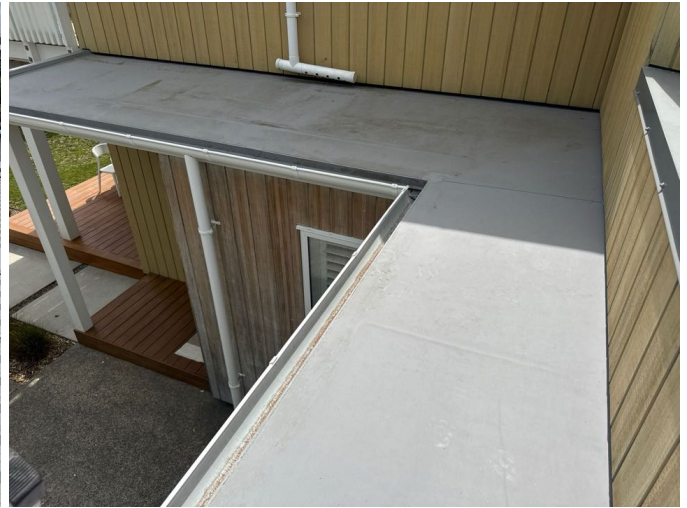
The waterproof membrane sections are intact and in good condition
