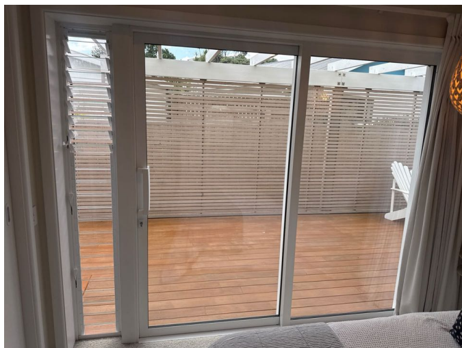
The louvre windows and sliding door are functioning well
