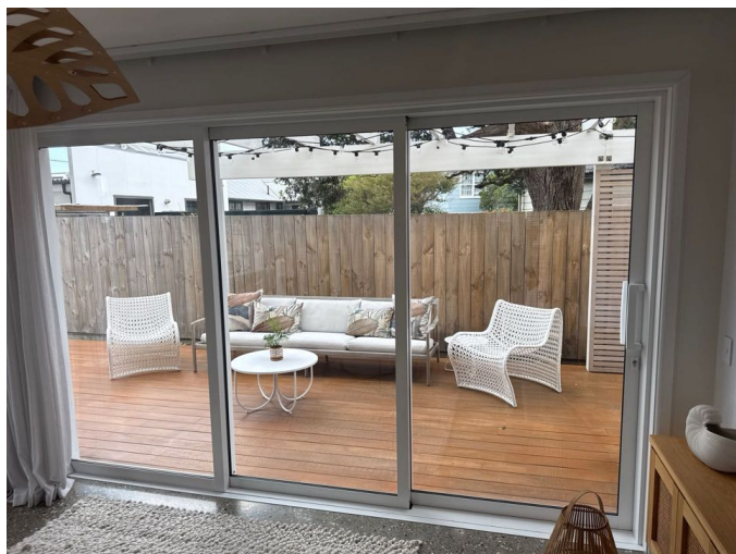
External doors are functioning well
