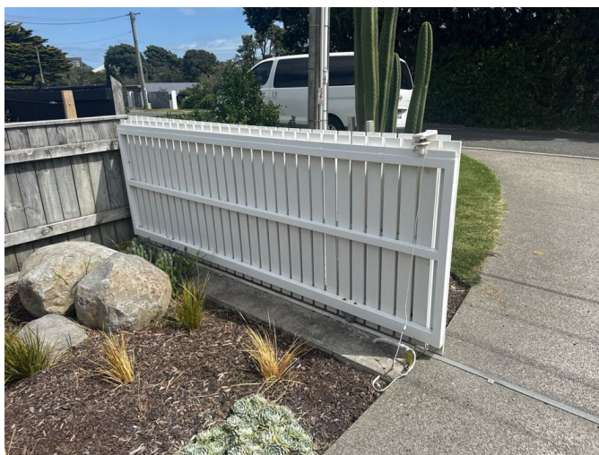
The electric gate to the driveway was not tested by T.H.I.S
