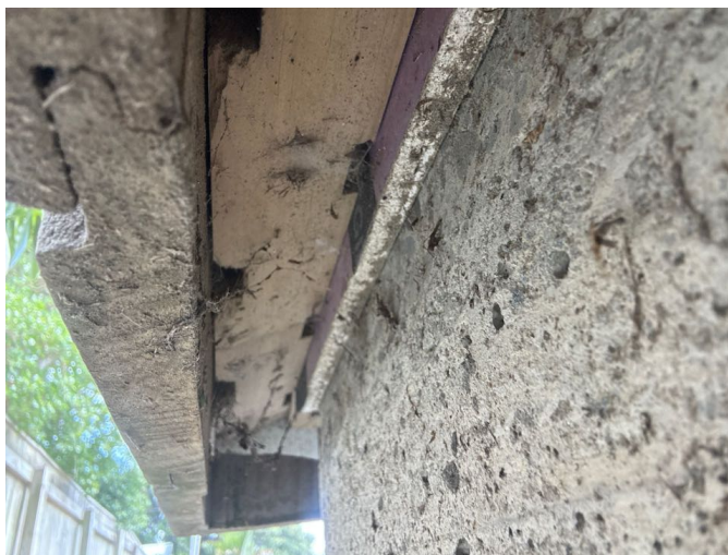
Cavity system detail noted. The cavity system is a modern detail that allows moisture to escape and ventilation to the back of the cladding.
