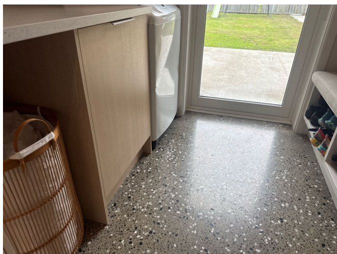
The cabinetry and concrete floor are in good condition
