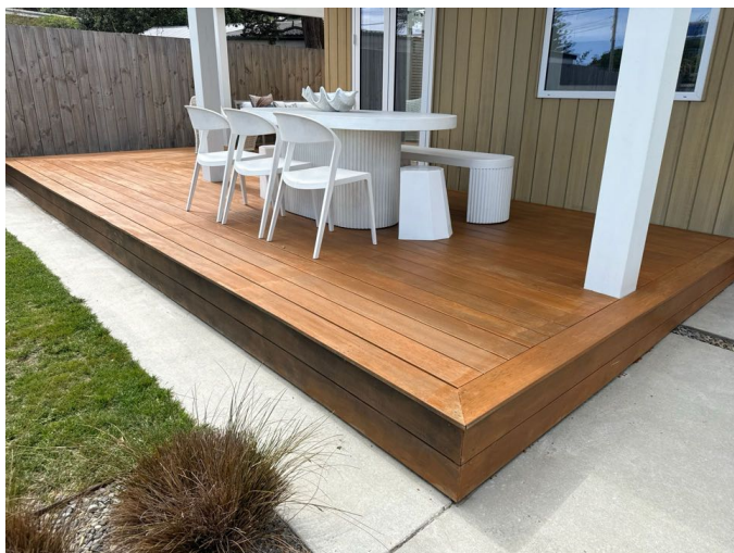
The low height timber deck has been finished to a good standard. No concerns found.
