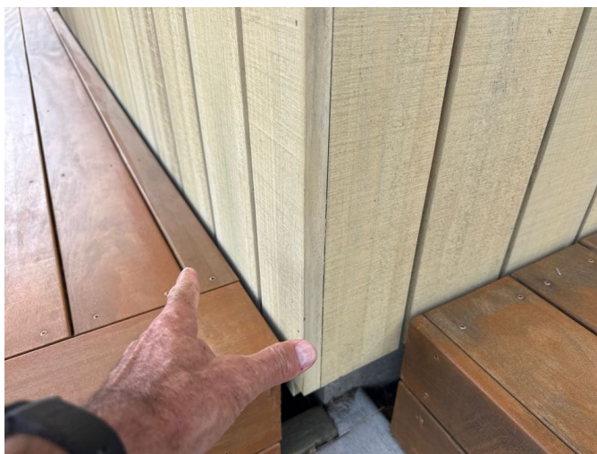
Good clearance between the decks and the cladding which will allow water to drain away.
