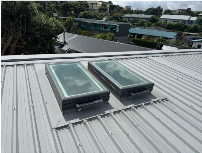
The skylights are effectively flashed and sealed
