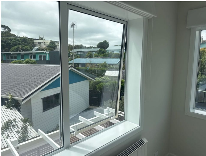
The windows are functioning throughout
