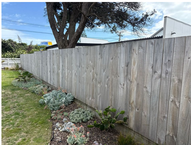
The perimeter fencing is solid and intact.
