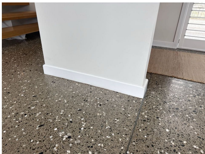
The concrete floor and wall linings are in good condition
