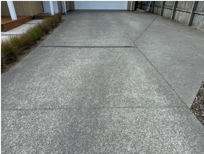
The driveway is well formed and in good condition
