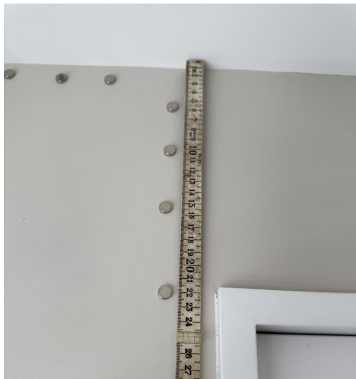
Photograph 4. Typical bracing panel fixing check.
