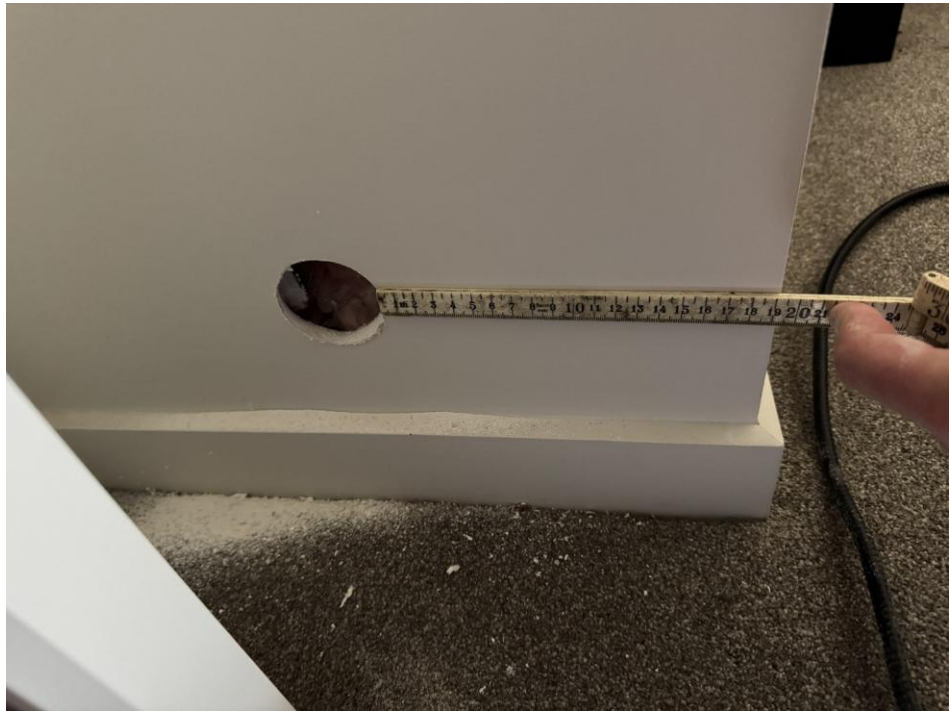
Photograph 3. Typical invasive investigation .
