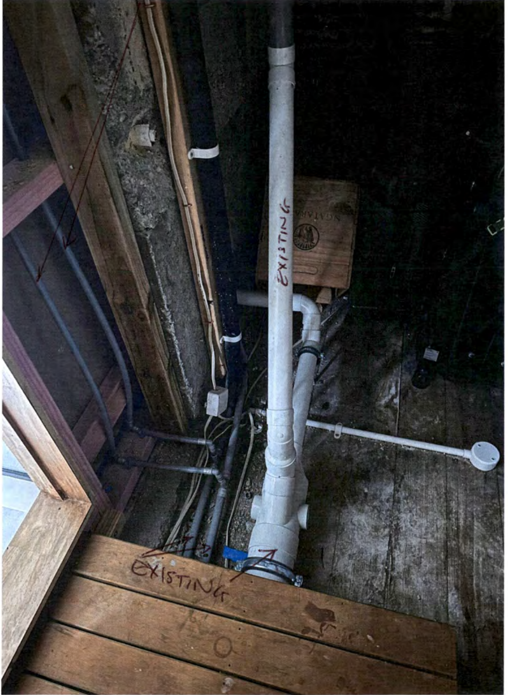
EXISTING SEWER + VENT PIPE.
