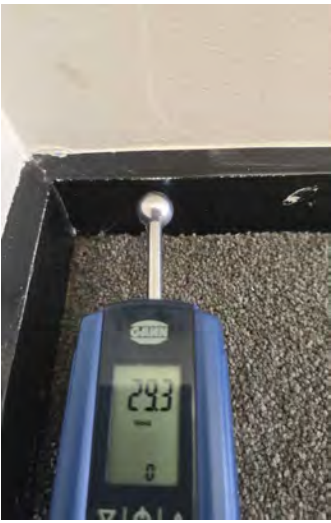
Behind the shower on the opposite side of the wall.
