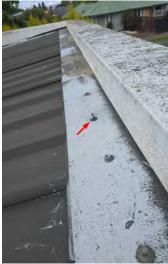
Popped nails along the ridge flashing.
