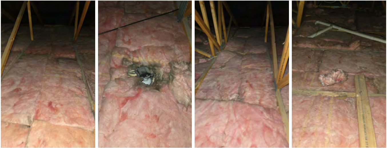
An example. The batts should be pulled away from the lights.
