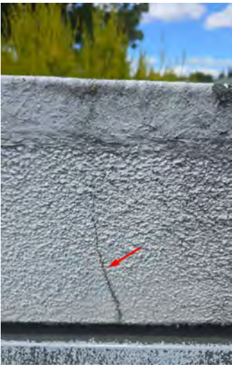
Minor cracking above the garage.
