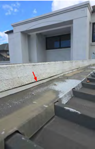
The plastic molding under the polystyrene has fallen down above the garage.
