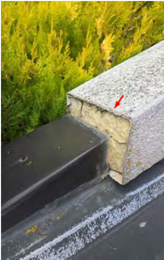
Missing flashing above the garage.
