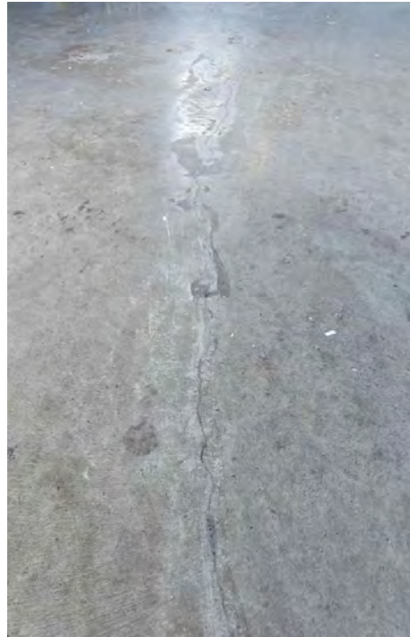
Evidence of repairs.
