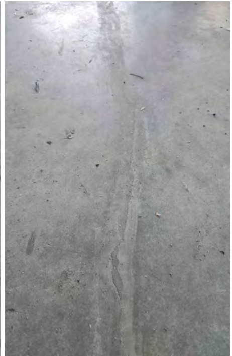
Evidence of repairs.
