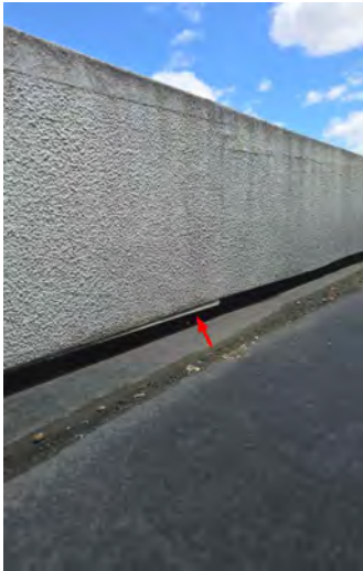
The plastic molding under the polystyrene has fallen down above the south side flat roof.
