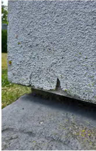
Minor cracking at the bottom of the pergola post.
