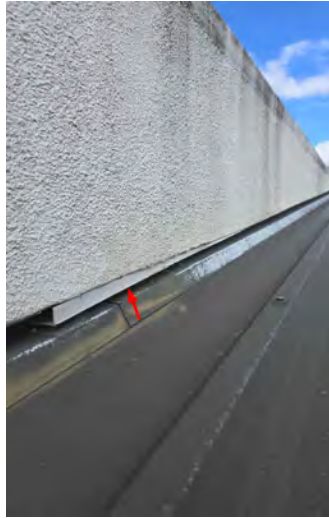
The plastic molding under the polystyrene has fallen down above the garage.
