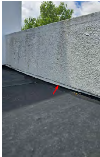
The plastic molding under the polystyrene has fallen down above the south side flat roof.
