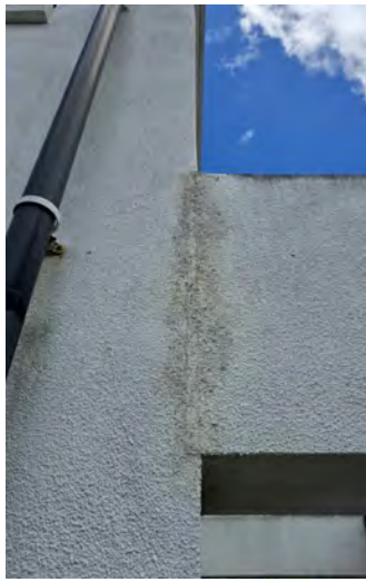
Evidence of repairs.
