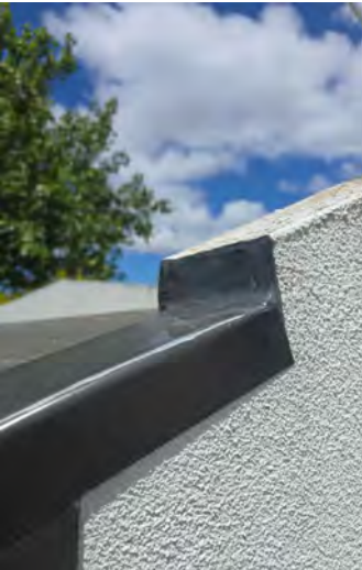
The plastic molding under the polystyrene has fallen down above the garage.
